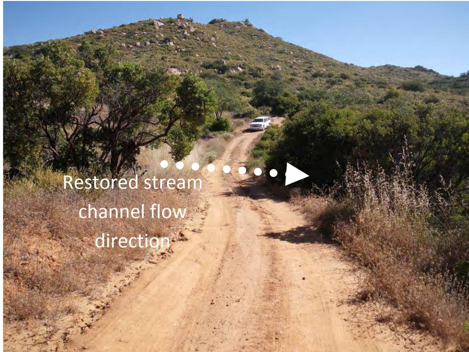
Figure C-21. View of existing road crossing at Site 11. Removal of road will re-connect the upstream and downstream reaches of this ephemeral stream channel, in addition to re-focusing the headwater drainage to the stream channel.
