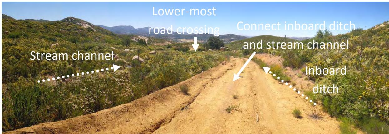
Figure C-12. At Site 1 looking down-gradient along the roadway with the stream channel running parallel to the left and an inboard ditch running on the right. The inboard ditch connects the abandoned road/ditch channel upstream to the ditch channel downstream.
