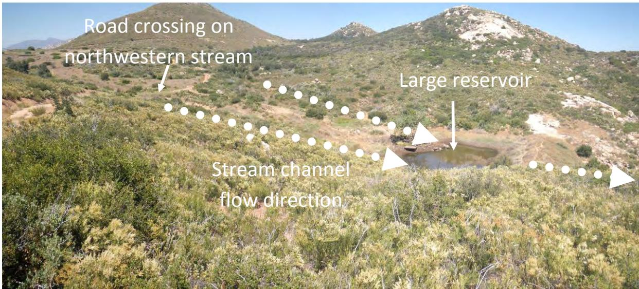
Figure C-25. Eastward view of the large reservoir, dam, road crossing, and northwestern and northeastern stream channels at Sites 2 and 3. Removal of road crossing and pond storage berms and lowering of the large reservoir dam will enhance hydrologic connectivity from the headwaters to the downstream of the large reservoir.
