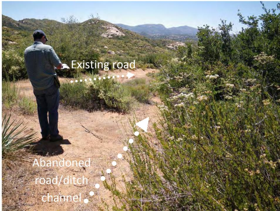
Figure C-11. At Site 1 looking downstream along abandoned road/ditch channel towards its confluence with the existing roadway. At the road, this channel continues along an inboard ditch.
