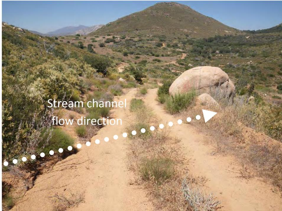
Figure C-18. View of existing road crossing (southwestern stream channel) at Site 2. Removal of road will re-connect the upstream and downstream reaches of this ephemeral stream channel.
