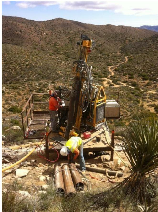
Micropile drilling at EP 225-1, Link 1.
