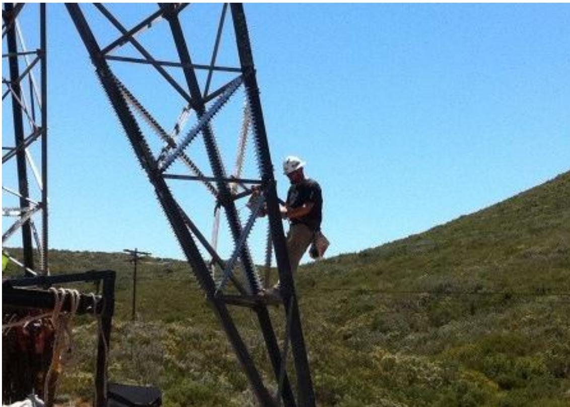
Installing anti-climbing guards at EP27-1. ([Link 2](#))
