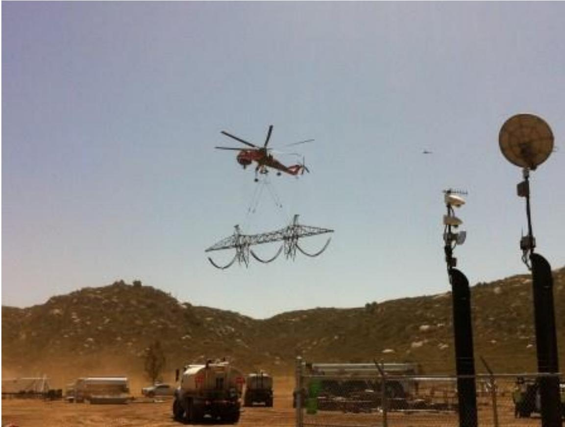
Aircrane flying tower bridge to Tower EP54. (Link 2)
