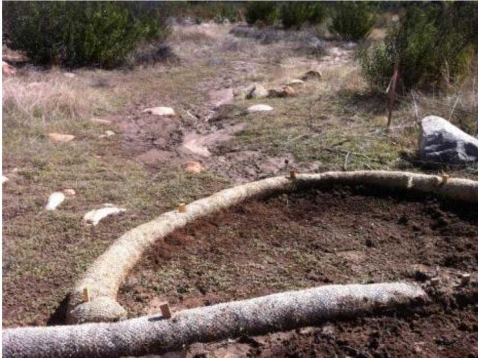
Breached BMPs with sediment going offsite at CP70-3. (Link 5)
