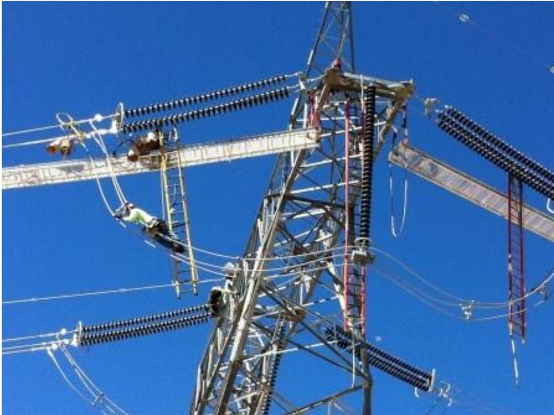
Installing jumpers at Tower EP200-3. (Link 1)
