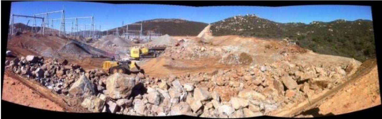
Rock being crushed for Class 2 base and select fill. (Link 3)
