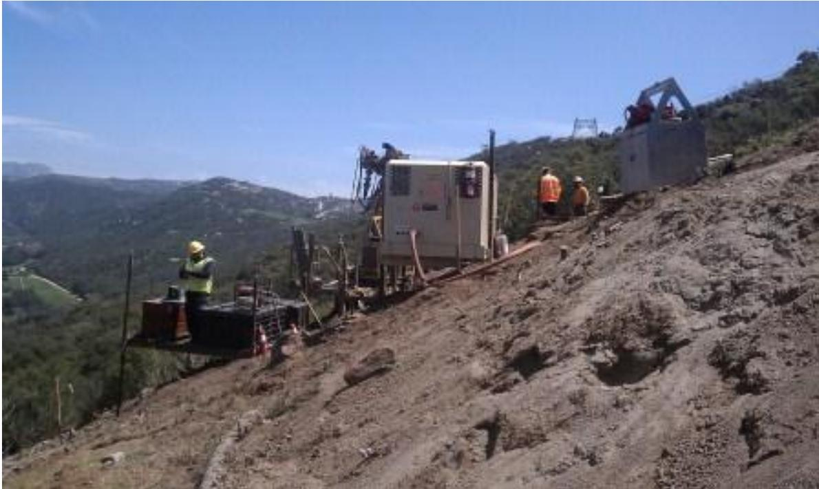
Micropile drilling at EP10-2, Link 2.
