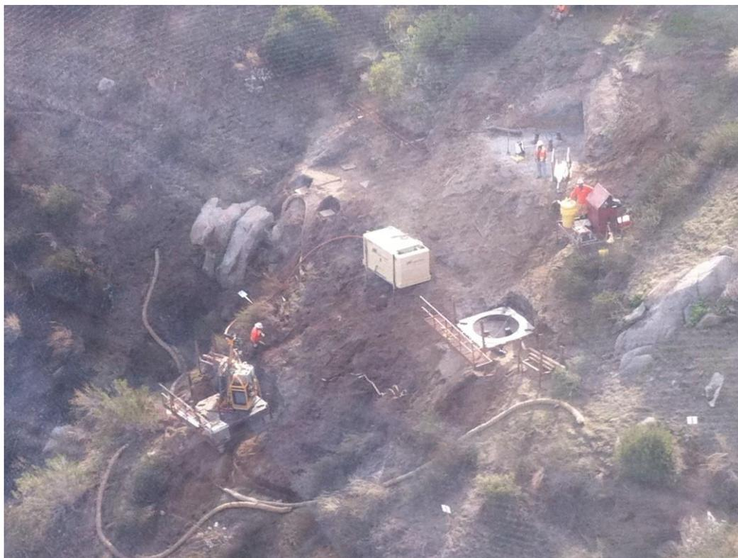
Micropile drilling operations at CP61-1.
