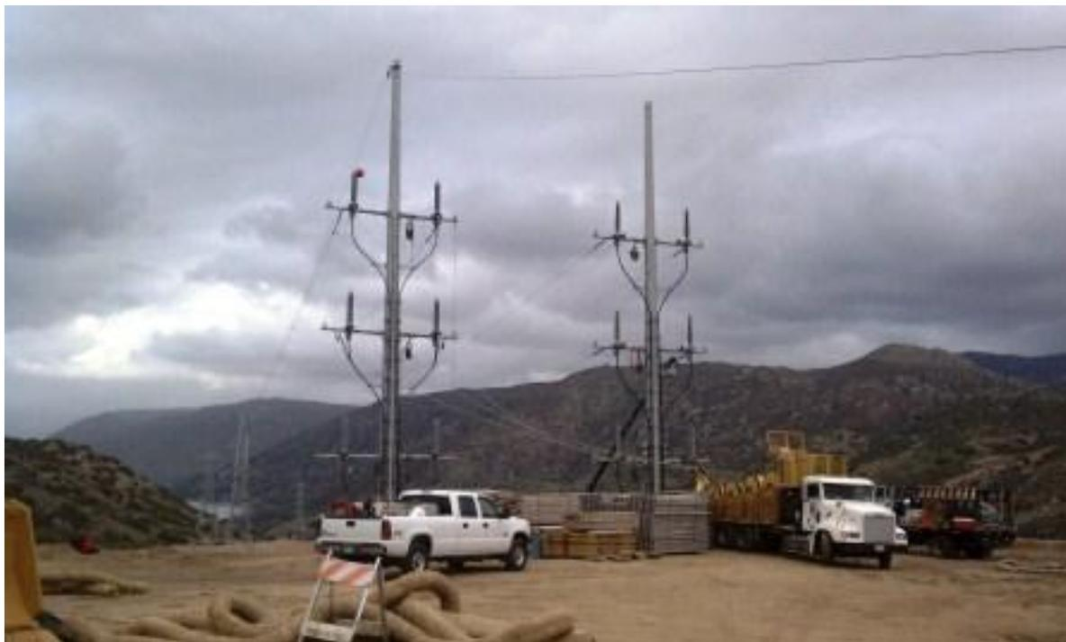
Wire pulling operations at transition structure CP88-1.
