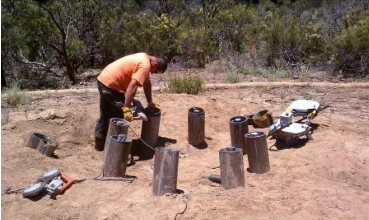
Trimming micropiles at EP 85-2, Link 2.
