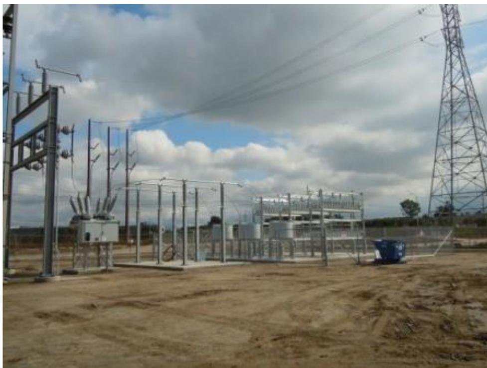
69 kV capacitor bank at South Bay Substation.
