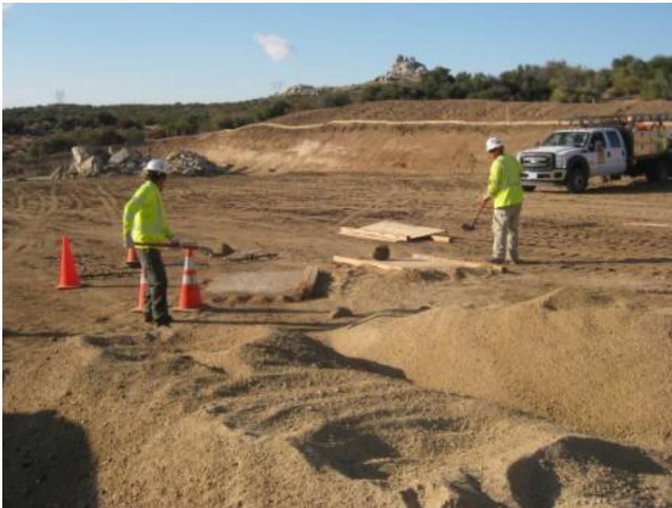
Crews covering foundations holes per the Mitigation Measures at EP219 pull site. (Link 1)
