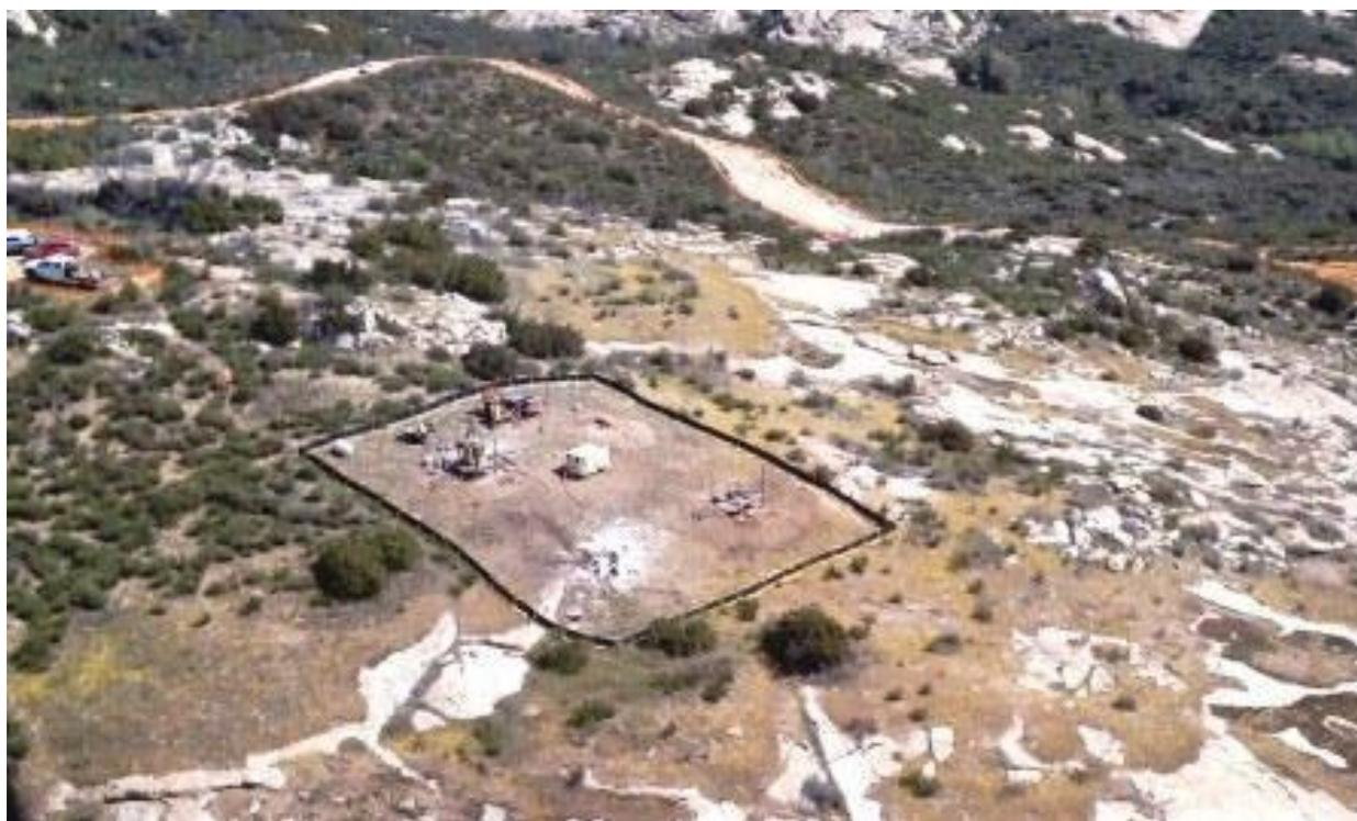
Helicopter view of micropile drilling at Tower EP50 with Arroyo Toad exclusionary fencing around the site. (Link 2)
