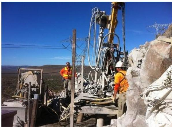
Photo 6: Micropile drilling at Tower EP 254-3, Link 1.
