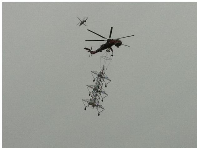
*Photo 35: Aircrane and KMAX helicopters during tower assembly activities in El Monte Valley.*
