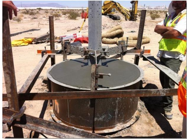
Photo 9: Conventional foundation pour at EP 336, Link 1.
