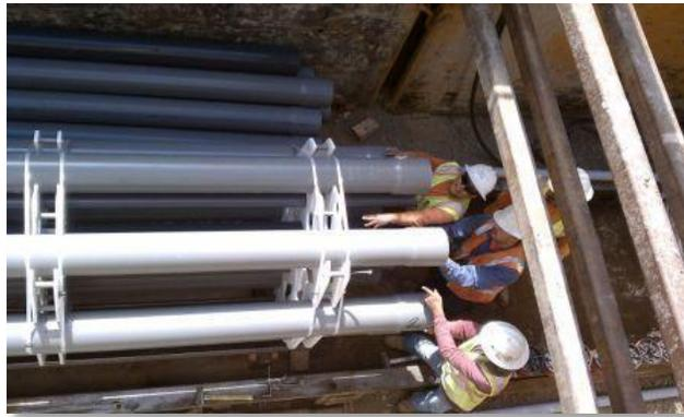
*Photo 21: Crews installing conduit at the jack-and-bore underneath Interstate 8, Link 4.*
