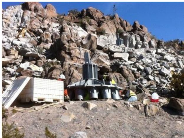
*Photo 4: Micropile cap work at EP 254-3, Link 1.*
