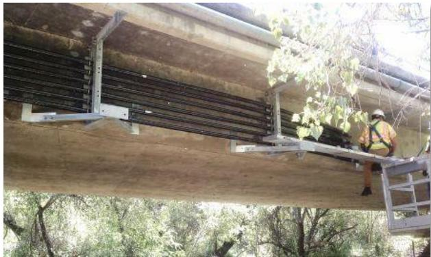
Photo 19: Attachments of Conduit to Viejas Bridge, Link 4.
