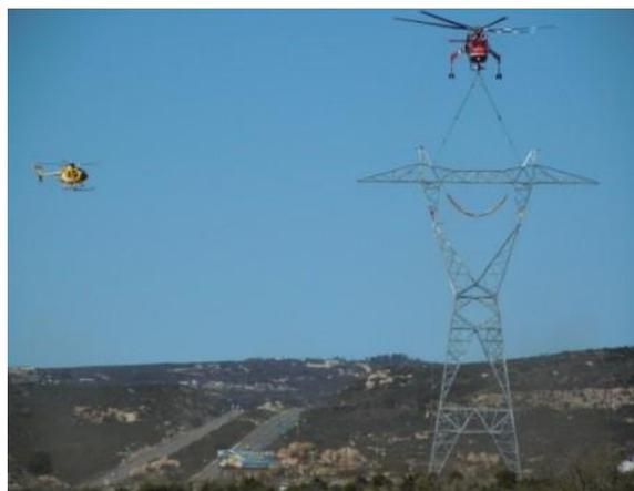
Photo 7: Aircrane is placing the bridge on EP 217, Link 1.
