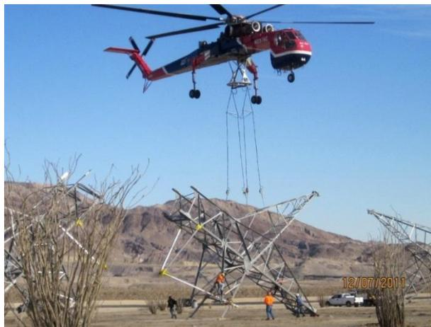
Photo 30: Aircrane tower pick at S2 Yard.
