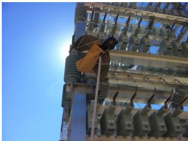
Photo 27: One of the various types of bird deterrents at Suncrest Substation, Link 3.
