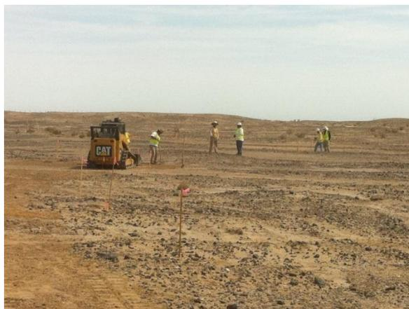
*Photo 8: Raking desert pavement at EP 341, Link 1.*
