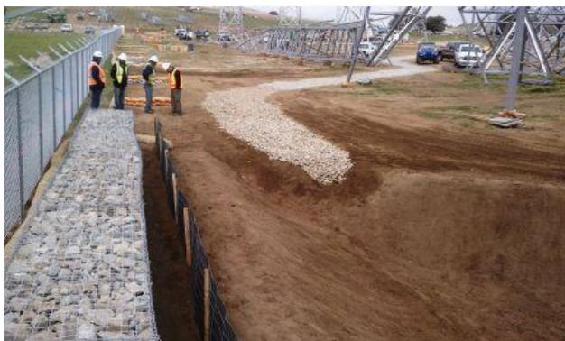
*Photo 34: Stormwater BMPs improved at the Bartlett-Hauser Yard, Link 2.*
