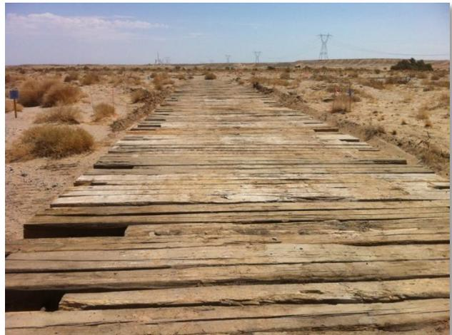
Photo 10: Temporary Douglas Fir mat access road over dry wash at EP 324, Link 1.
