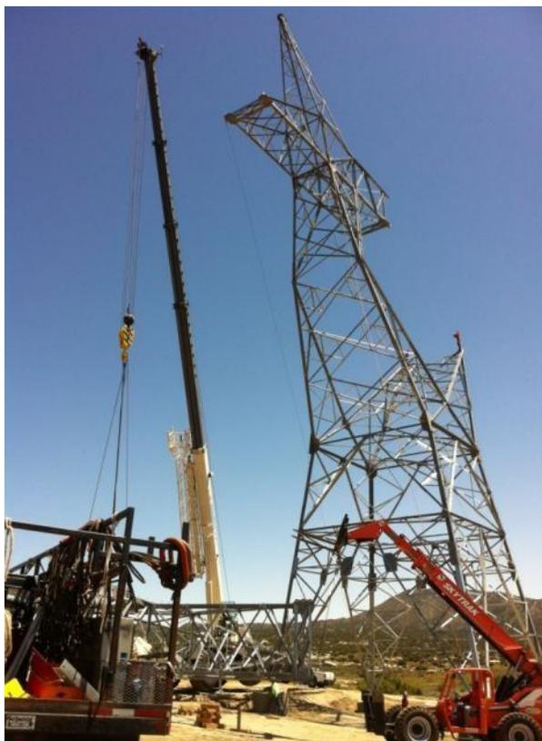
Photo 2: Conventional tower assembly at EP 210, Link 1.
