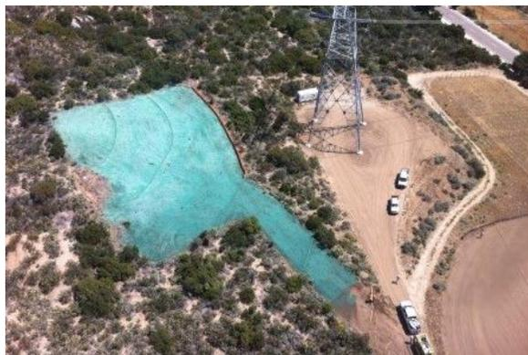
*Photo 40: Hydromulching at EP 89-1 pull site, Link 2.*
