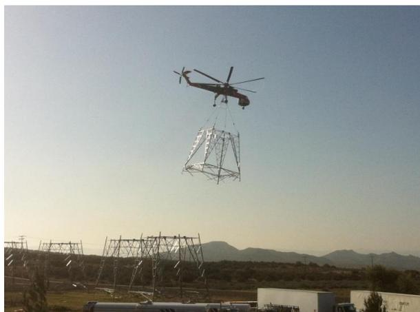
Photo 3: Skycrane flying with tower to EP 209, Link 1.
