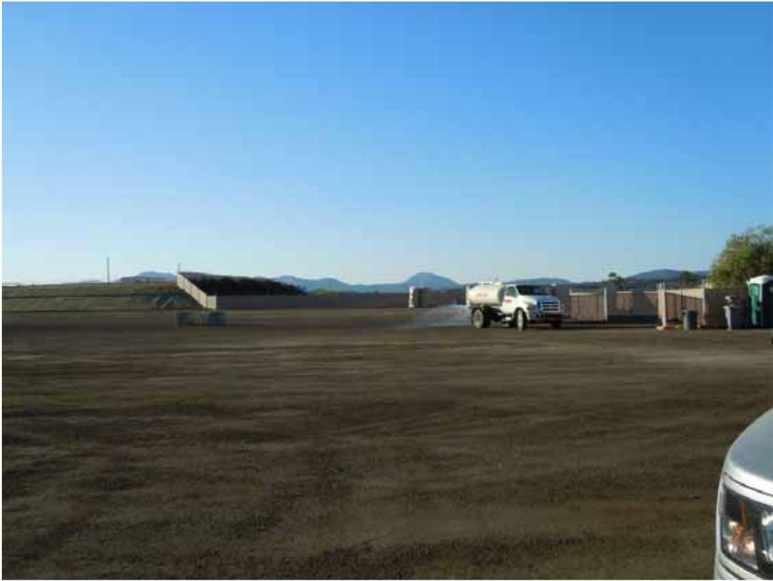
**Figure 5:** Water truck performing dust control activities at the Alpine Laydown Yard.
