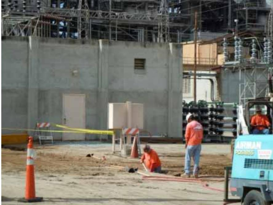
**Figure 1:** Trenching continues at the South Bay Substation.
