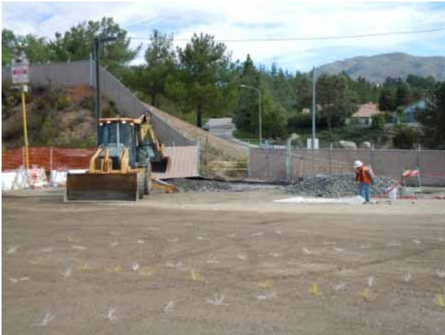
**Figure 2:** Construction exit being installed at the PAR portion of the Alpine Construction Yard.
