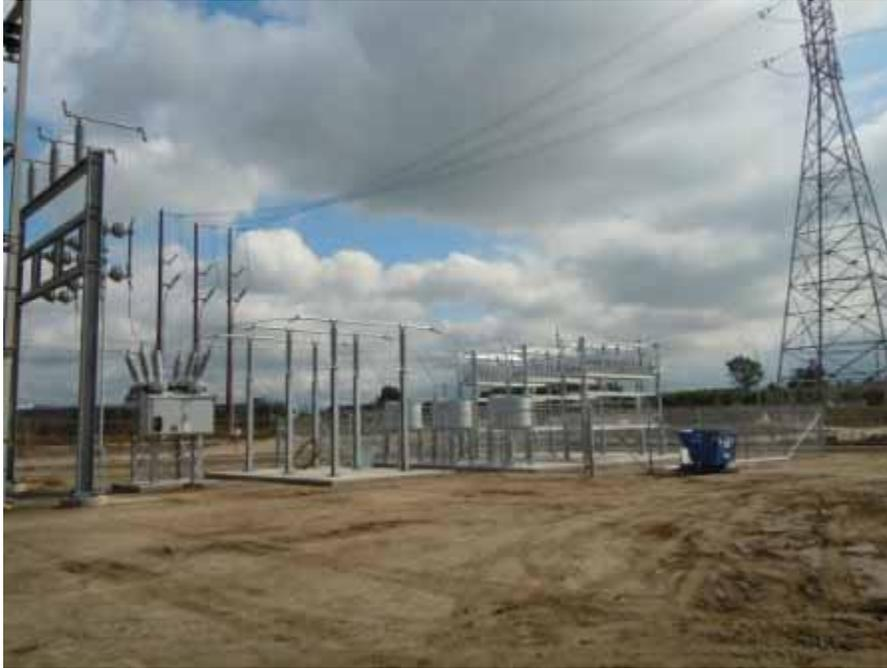
**Figure 1:** 69 kV capacitor bank at South Bay Substation.
