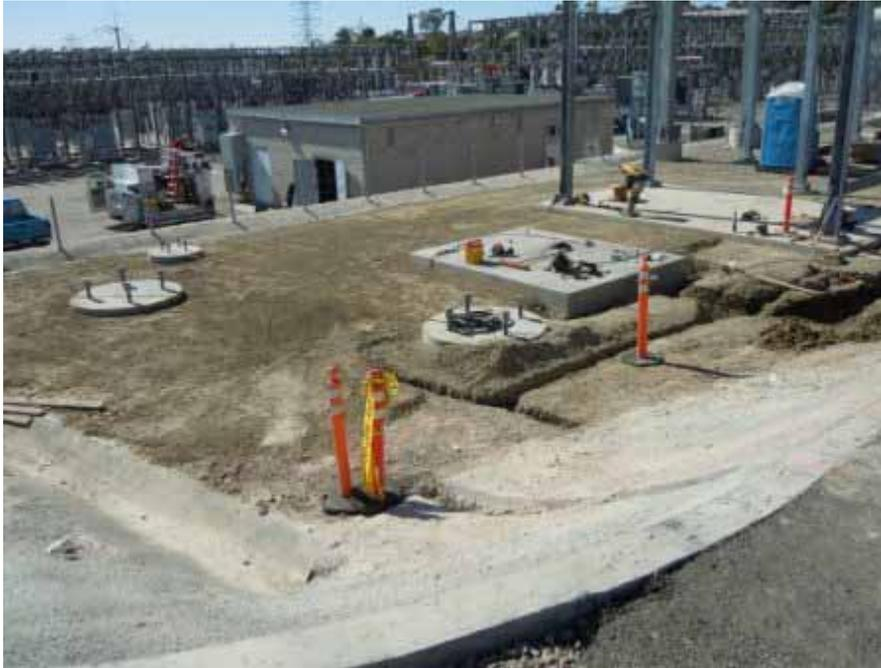
**Figure 1:** San Luis Rey Substation foundation installation.
