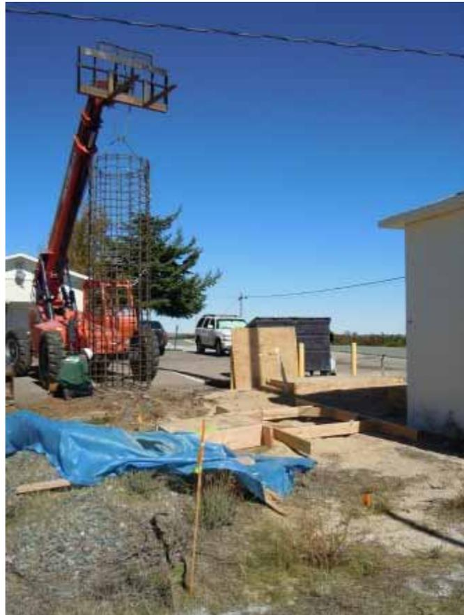
**Figure 4:** Rebar cage installation at the White Star Telecommunication site.
