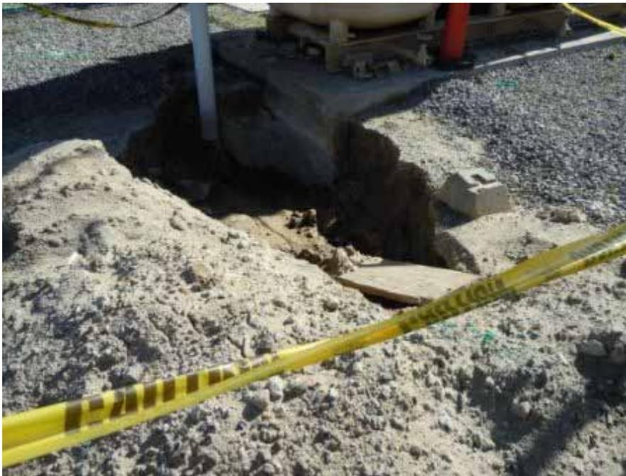
**Figure 2:** Ramping of an excavation at the Encina Substation.
