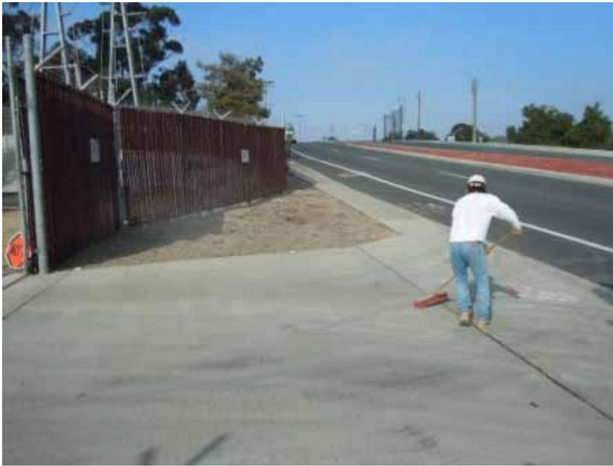
**Figure 3:** Crew member sweeping minor trackout at the San Luis Rey Substation.
