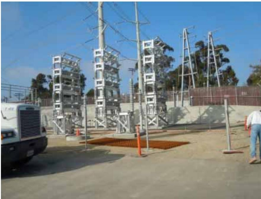
**Figure 2:** Fence and concrete pad installation at San Luis Rey Substation.
