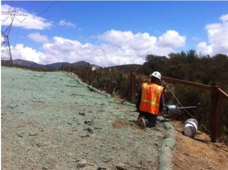
**Figure 1:** Hydromulching and fence installation at EP124/125 pull site. (Link 2)
