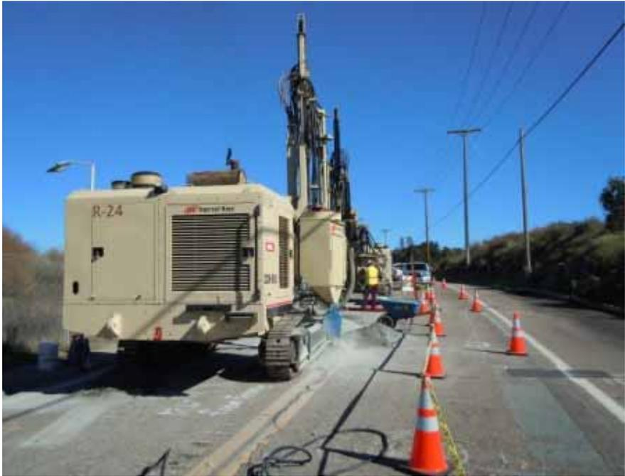
**Figure 2:** Drilling along Alpine Boulevard in preparation for vault excavation, Link 4.
