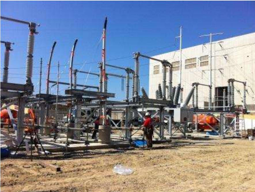
Figure 2: Steel assembly at Encina Substation.
