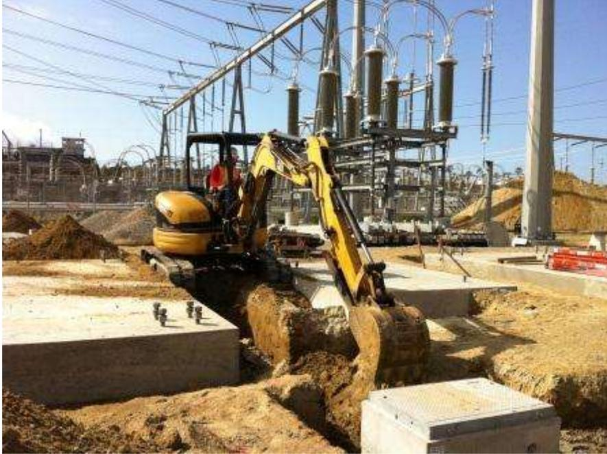
Figure 1: Digging trenches for conduit at Encina Substation.
