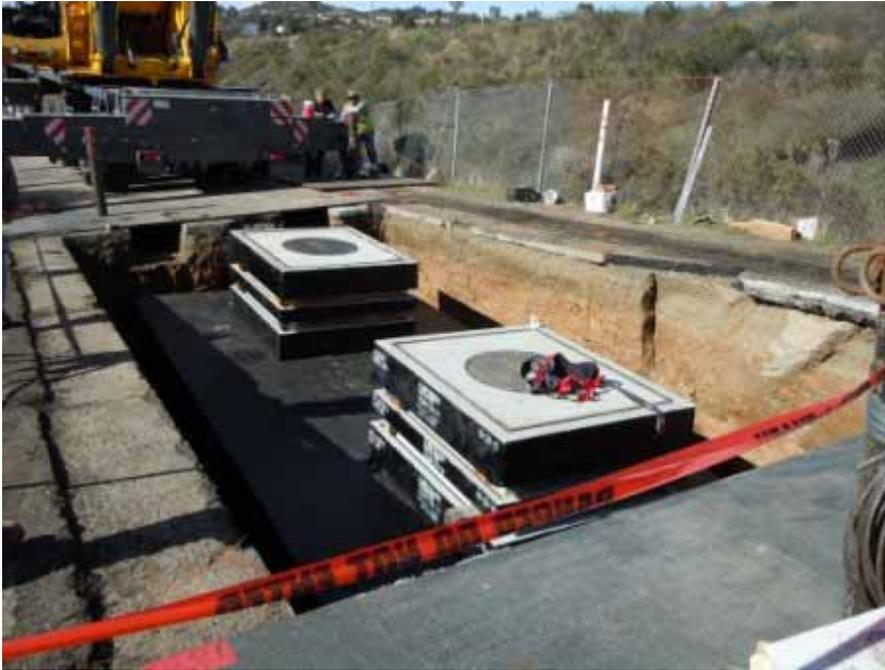
**Figure 2:** Manholes after the vault installation along Alpine Boulevard, Link 4.
