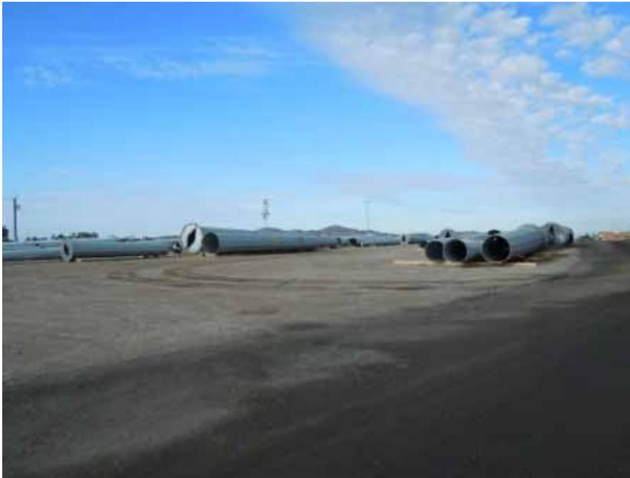
**Figure 4:** Monopole storage at the Alpine Construction Yard.
