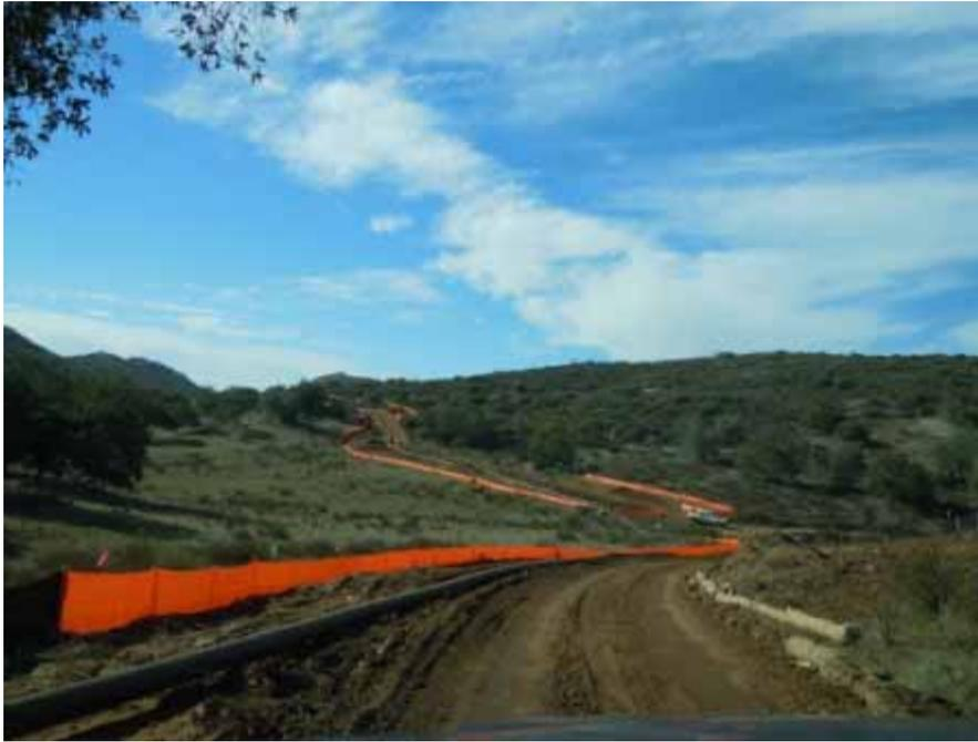
**Figure 3:** Vegetation clearing, rough grading and waterline installation at the Suncrest Substation.
