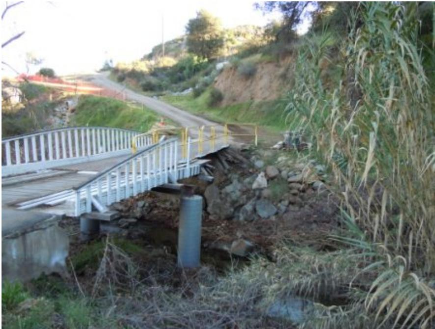
**Figure 2:** Bauer Property Bridge that was damaged by non-Sunrise related SDG&E operation & maintenance crews.
