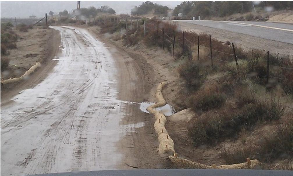
**Figure 4:** SWPPP installation during rain event on access road near Tower EP 214, Link 1.
