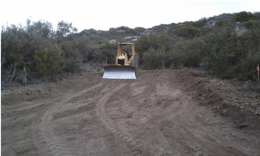
**Figure 1:** Grubbing completed at Tower EP 85, Link 2.
