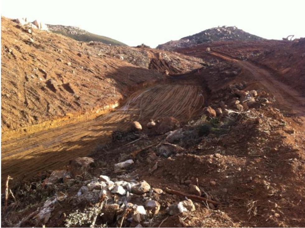
**Figure 5:** Sediment basin construction, Link 3.
