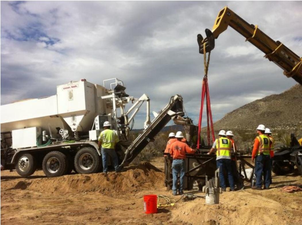
**Figure 2:** Foundation pouring at EP 244, Link 1.
