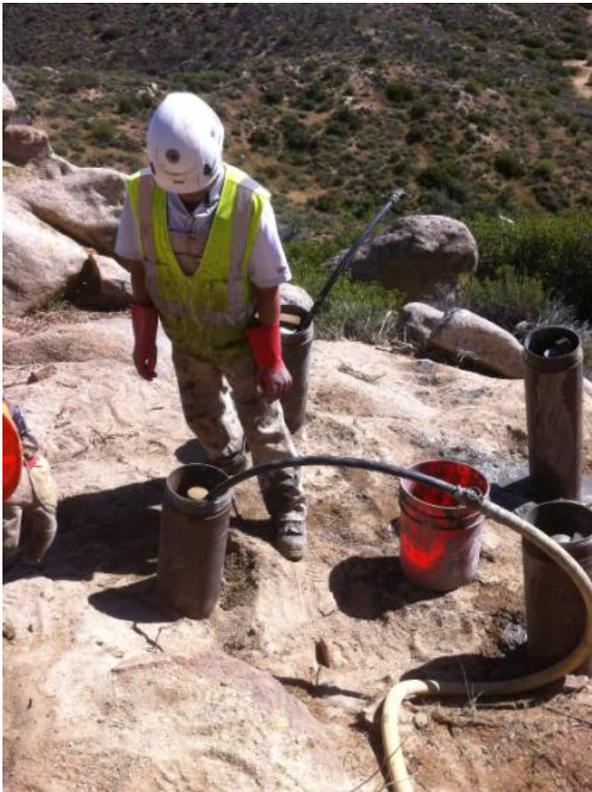
**Figure 1:** Micropile grouting at EP 225-1, Link 1.
