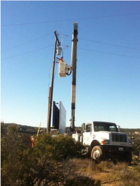
**Figure 2:** 12 kV relocation along McCain Valley Road, Link 1.
