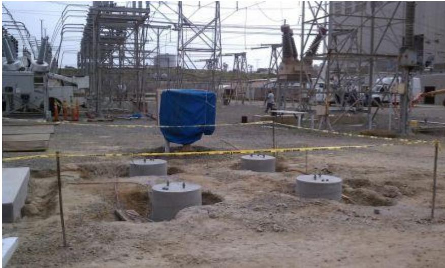
**Figure 7:** Footers poured at Encina Substation.
