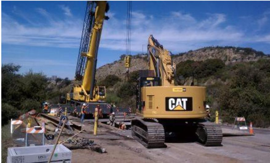
**Figure 3:** Vault being set, Link 4.
