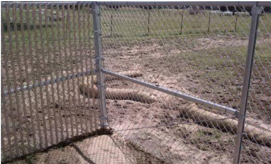
**Figure 6:** Stormwater BMPs breached at the Bartlett-Hauser Construction Yard, Link 2.
