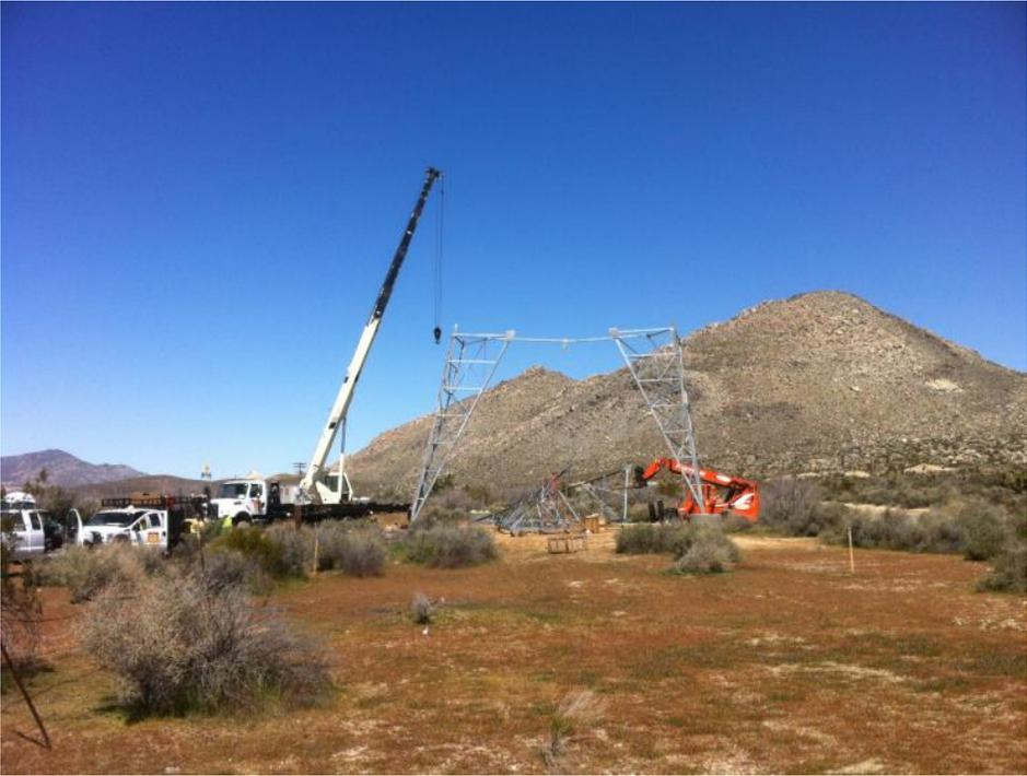
**Figure 1:** Conventional structure assembly at EP 243, Link 1.
