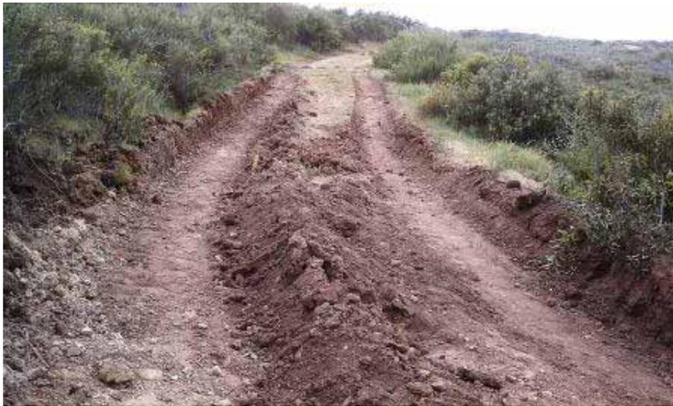
**Figure 6:** Ruts created by excavator on 69 kV, Link 5.
