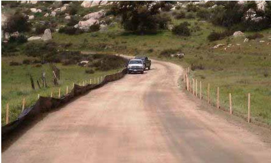
**Figure 9:** Silt/wildlife exclusionary fence installation along access road to Kreuzkamp Construction Yard, Link 2.
