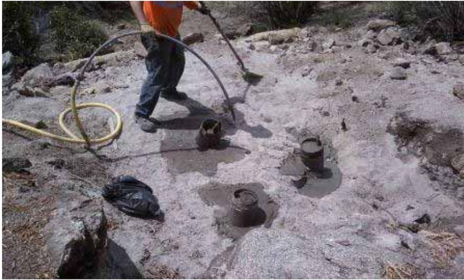
**Figure 1:** Micropile grouting at Tower EP 81, Link 2.
