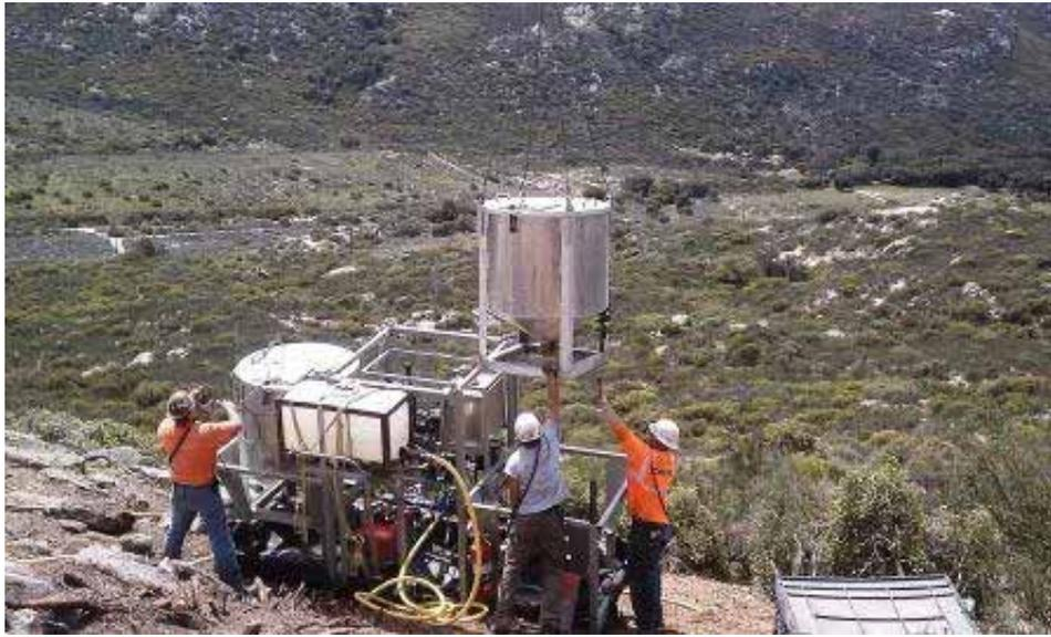
**Figure 3:** Crew securing new container of grout during helicopter delivery, Tower EP 81, Link 2.
