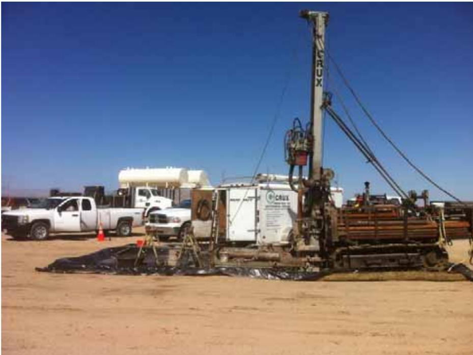
**Figure 2:** Micropile soil boring at EP330, Link 1.
