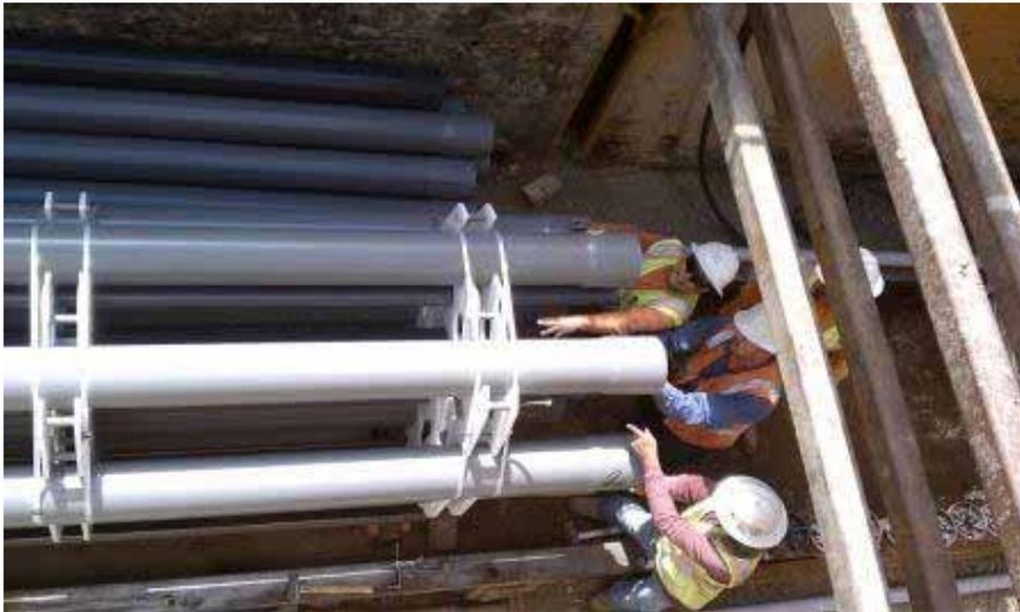
**Figure 4:** Crews installing conduit at the jack-and-bore underneath Interstate 8, Link 4.
