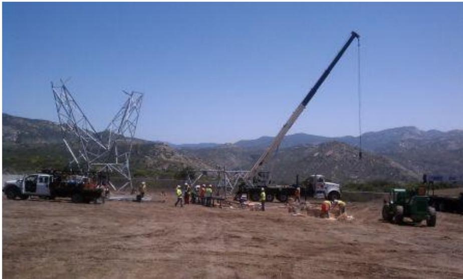
**Figure 6:** Tower assembly at SWAT Construction Yard, Link 2.
