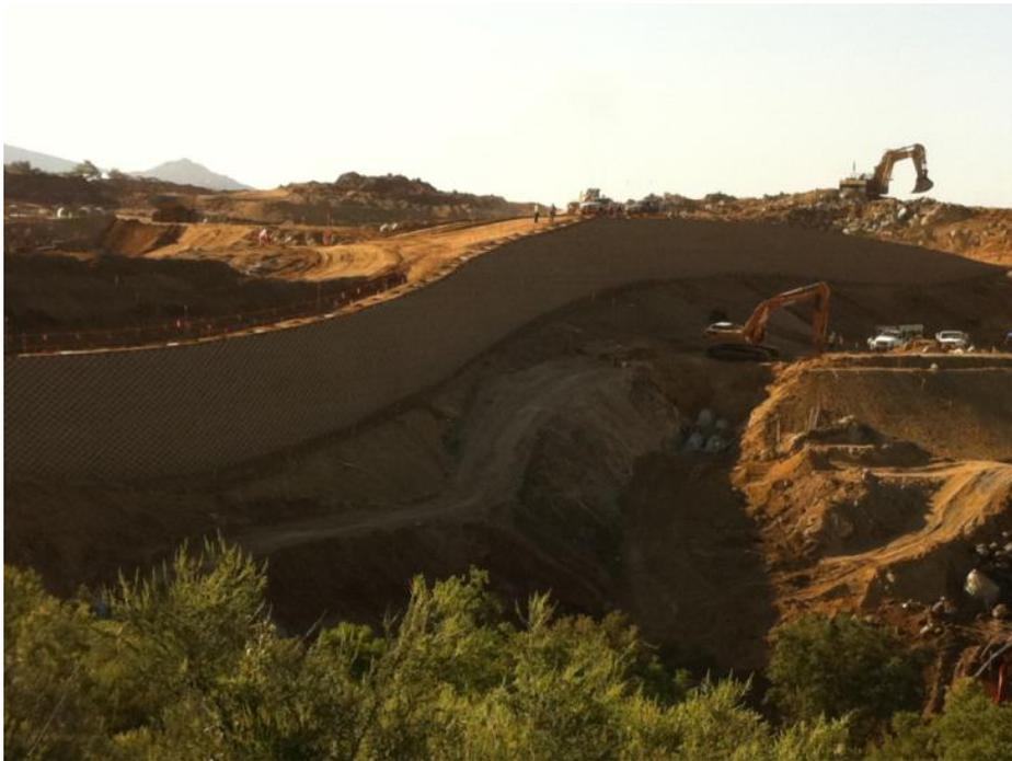
**Figure 5:** Completed northern soil retention wall at Suncrest Substation, Link 3.
