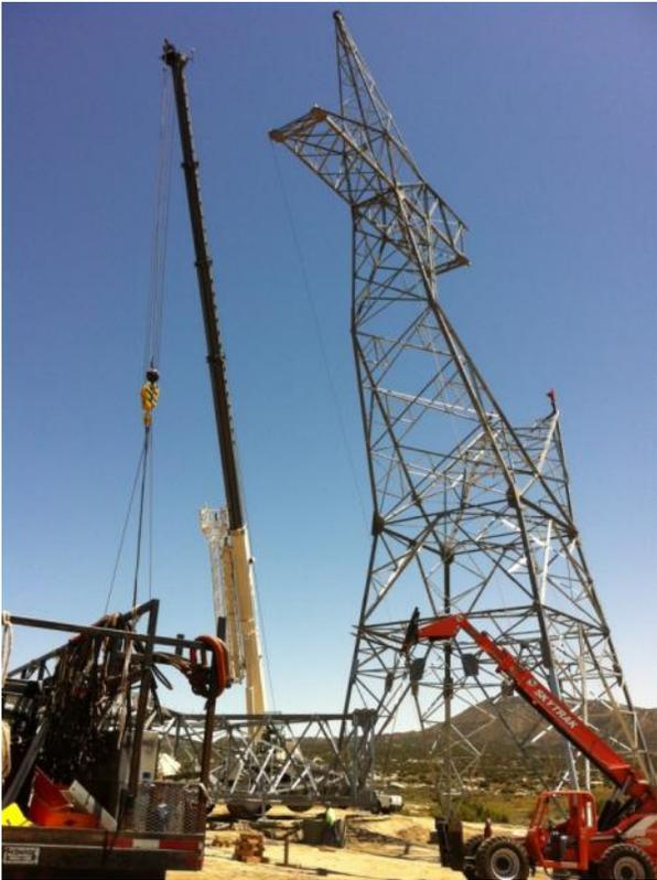
**Figure 1:** Conventional tower assembly at EP210, Link 1.
