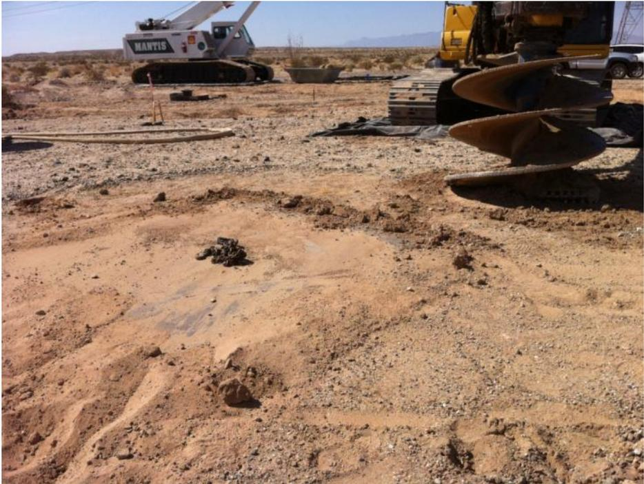
**Figure 2:** Steel plate with appropriate soil mounded around edges at EP337, Link 1.
