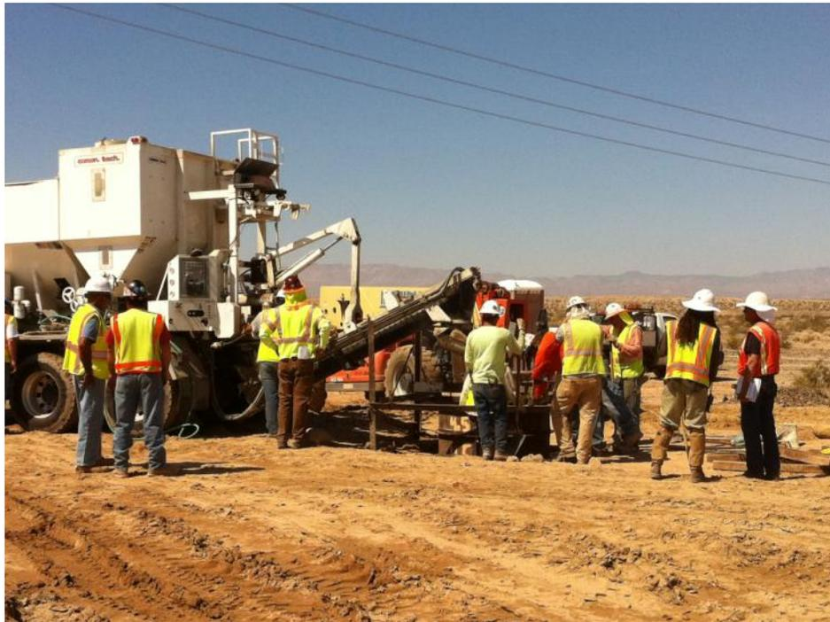
**Figure 3:** Conventional foundation pouring at EP338, Link 1.
