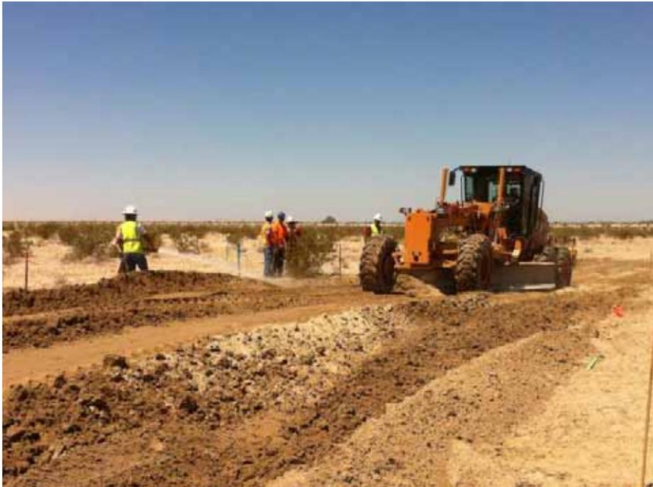
**Figure 2:** Grading EP362-1-N, Link 1.
