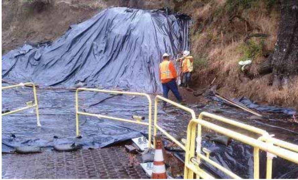
**Figure 1:** Crews hand digging pole sites for noise blanket installation at Bauer Bridge, Link 4.
