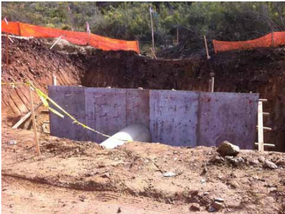
**Figure 6:** Culvert installation along BBTT, Suncrest Substation, Link 3.
