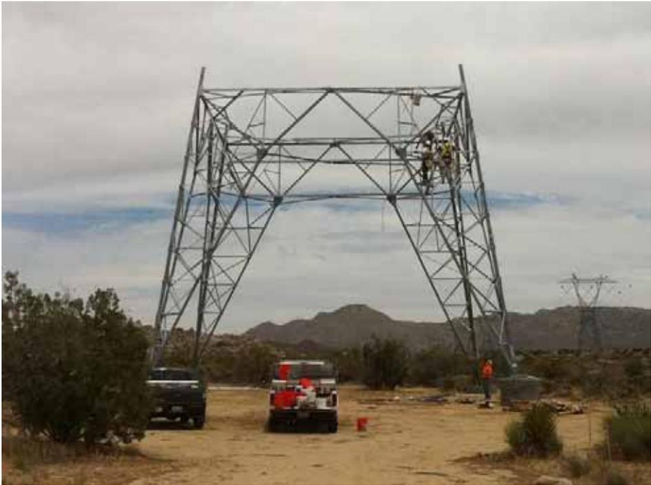
**Figure 1:** Conventional tower assembly at EP244, Link 1.
