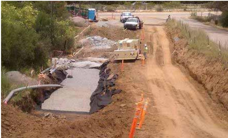
**Figure 4:** Grading and soil stabilization at Loritz Property, Link 4.
