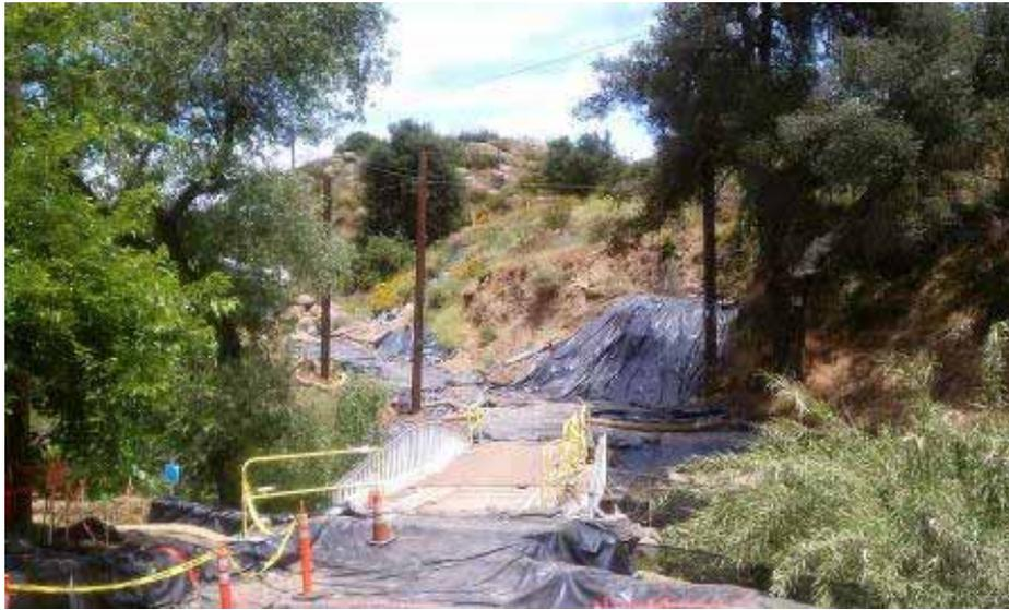
**Figure 3:** Poles for acoustic blankets were delivered and installed at Bauer Bridge, Link 4.
