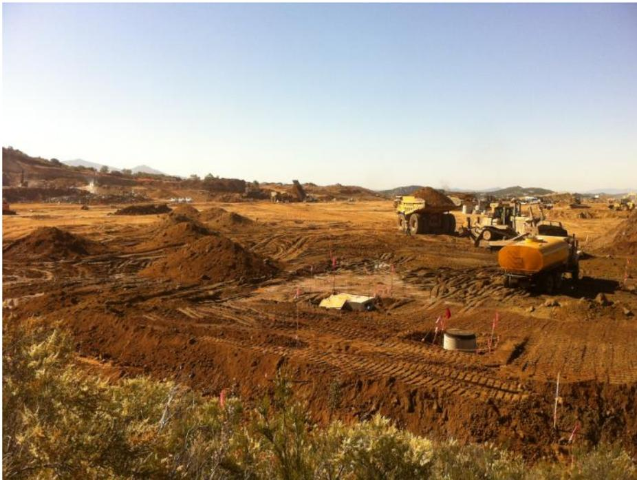
**Figure 10:** Bringing northwestern corner of substation pad to final grade, Suncrest Substation, Link 3.
