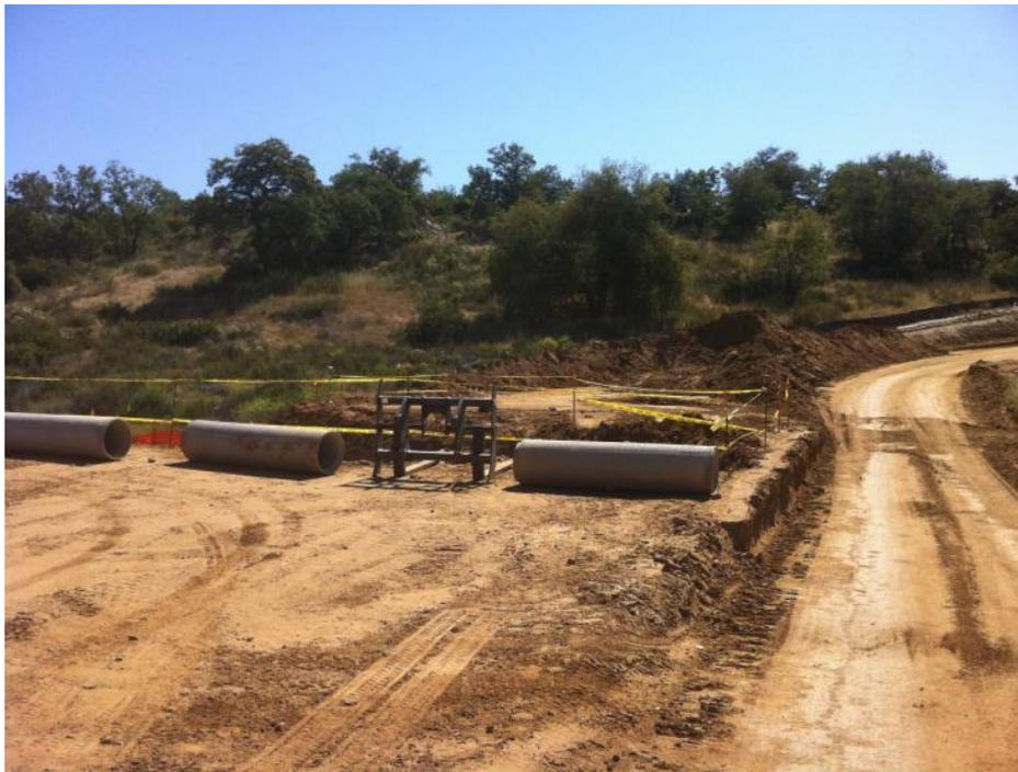
**Figure 8:** Culvert installation near Smith property, Suncrest Substation, Link 3.
