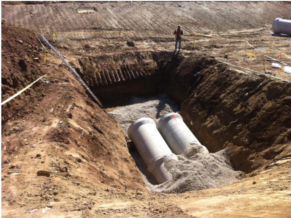
**Figure 9:** Installation of the permanent drainage system in the southern portion of the pad, Suncrest Substation, Link 3.
