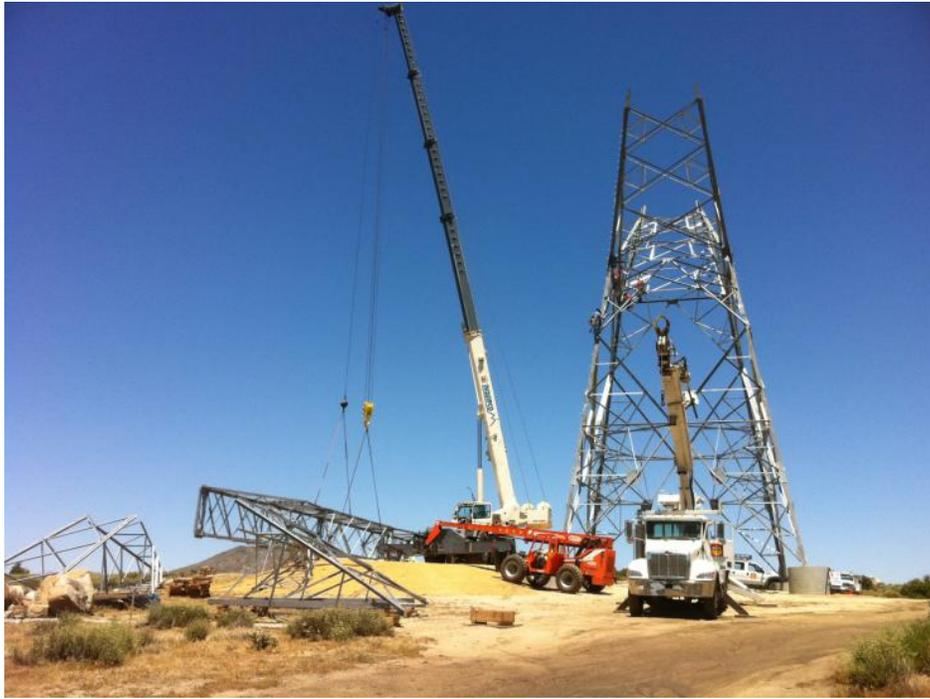
**Figure 1:** Conventional tower assembly at EP211, Link 1.
