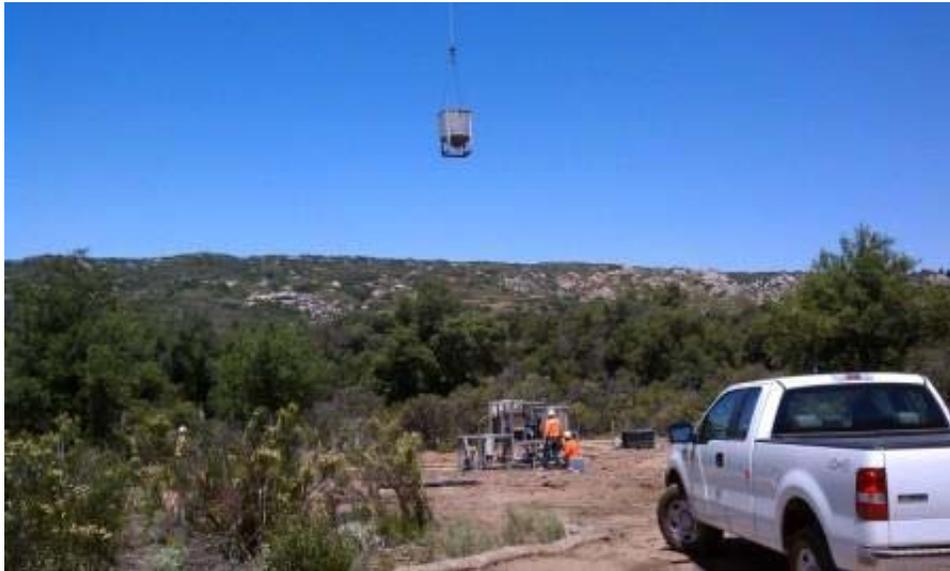
**Figure 3:** Helicopter delivery of grout at EP 85-1, Link 2.
