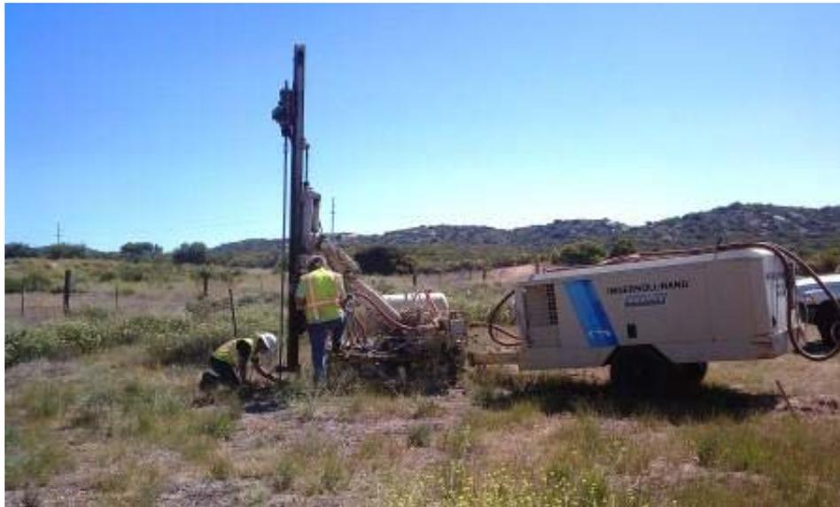
**Figure 2:** Micropile test drilling at EP 90-1, Link 2.
