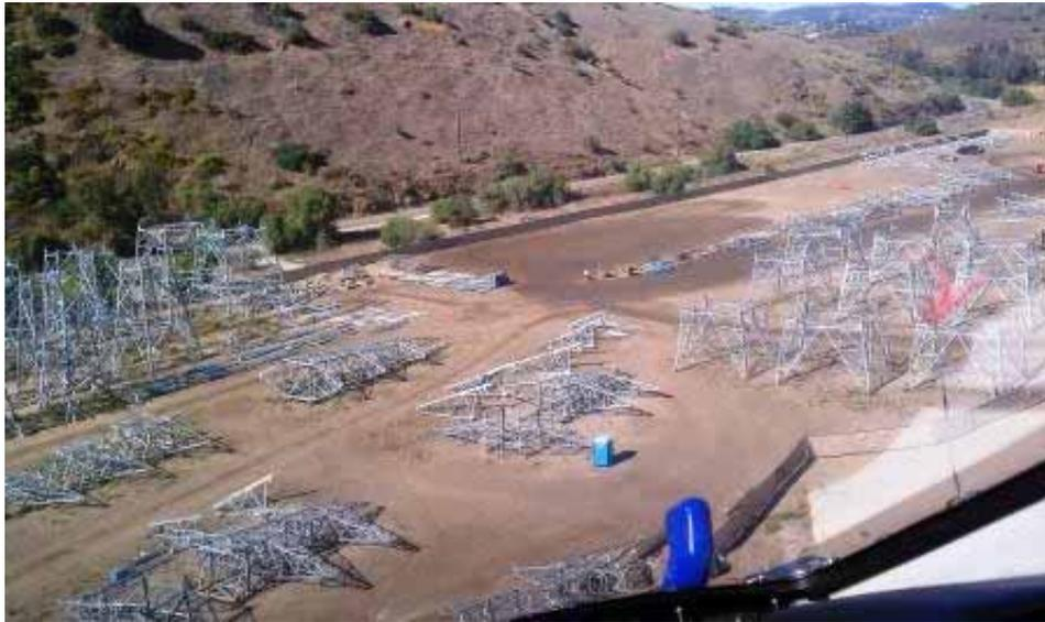
**Figure 7:** Helicopter view of Helix Construction Yard, Link 5. Note that landing area has been watered for dust control.
