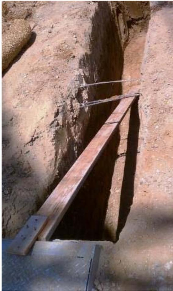
**Figure 9:** A wildlife escape ramp in a conduit trench at Encina Substation. The biologist reported a mouse used this ramp to escape after falling in the trench during construction.
