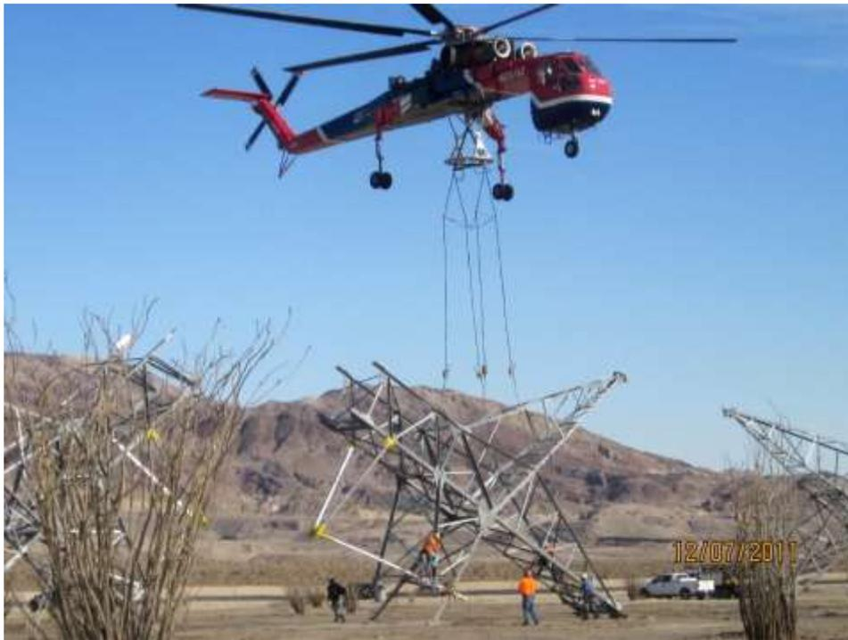
**Figure 9:** Air crane tower pick at S-2 Construction Yard. (Link 1)
