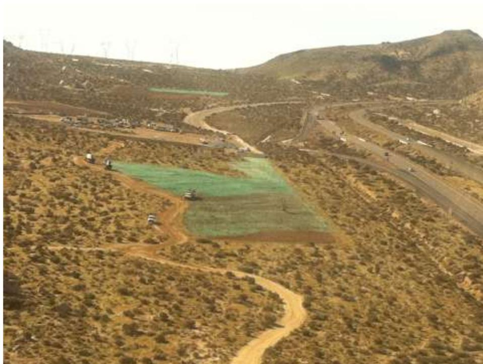
**Figure 4:** Hydromulch application to the lower section of Fromm Yard. The fenced area will remain. (Link 1)
