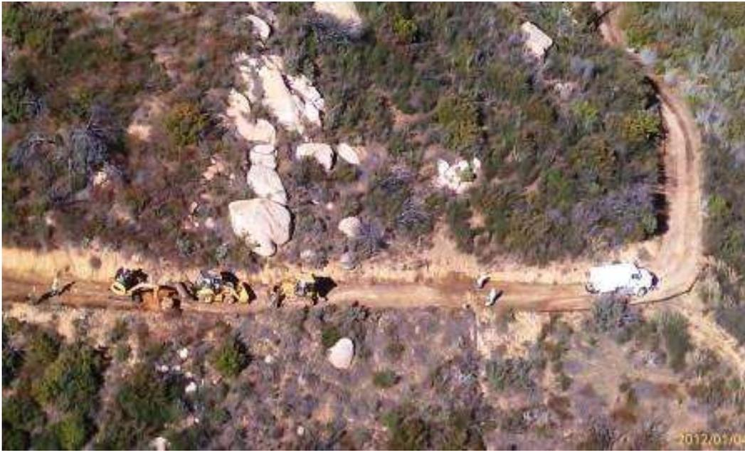
**Figure 3:** Road construction and boulder removal on USFS access road near EP36. (Link 2)
