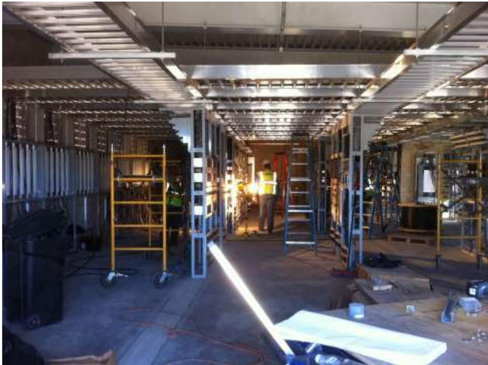
**Figure 5:** Starting wiring activities in the control house at Suncrest Substation. (Link 3)
