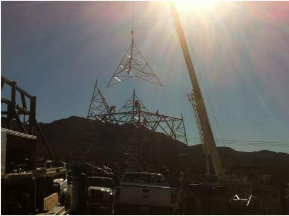
**Figure 2:** Conventional tower assembly at EP252-1. (Link 1)
