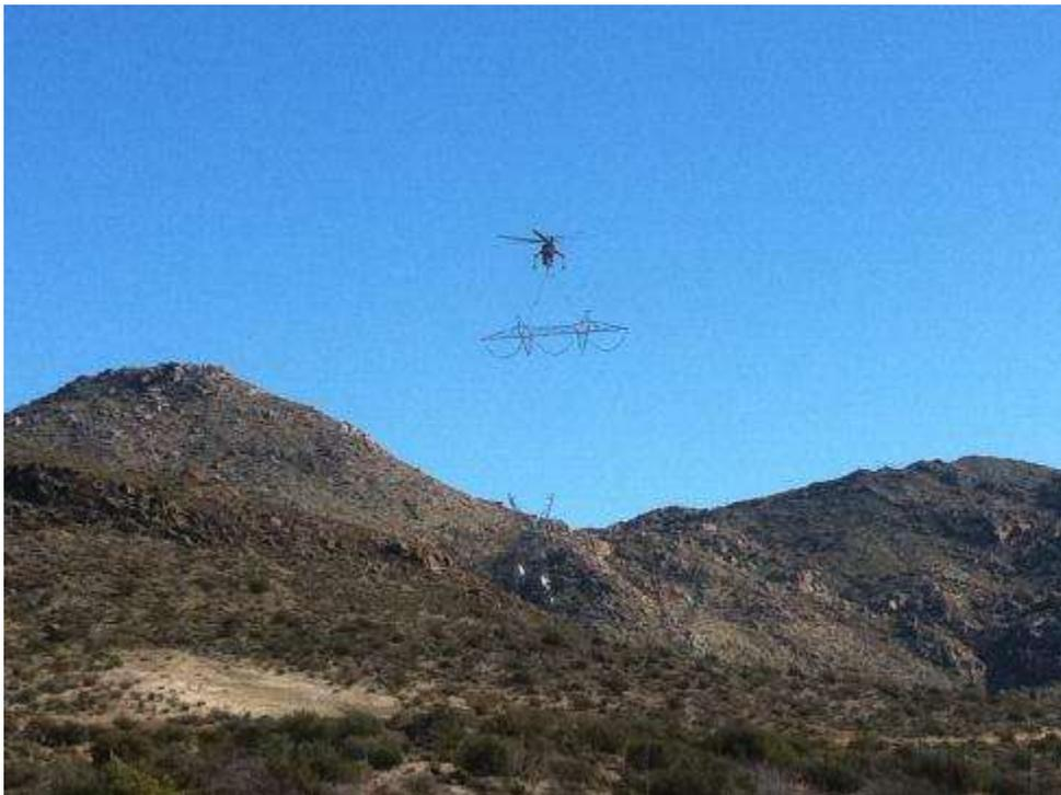
**Figure 4:** Aircrane setting bridge at EP253-3. (Link 1)
