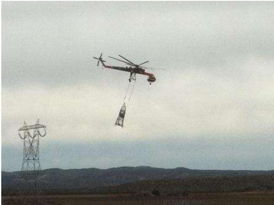
**Figure 12:** Air crane flying tower structures out of JVR Yard. (Link 1)
