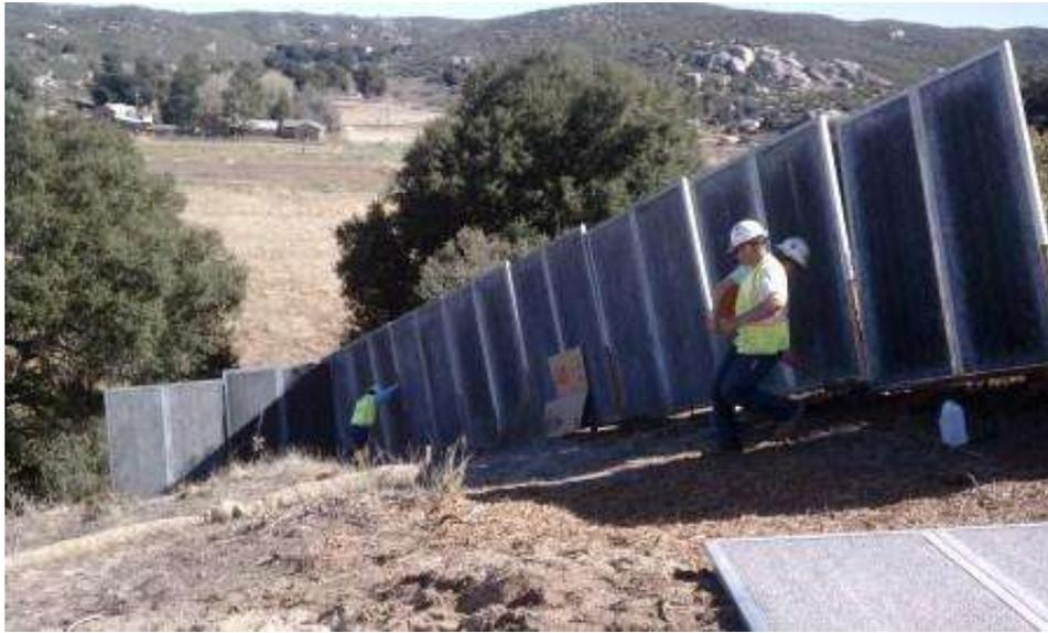
**Figure 3:** Construction of a sound wall at EP119. (Link 2)
