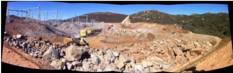
**Figure 10:** Rock being crushed for Class 2 base and select fill. (Link 3)
