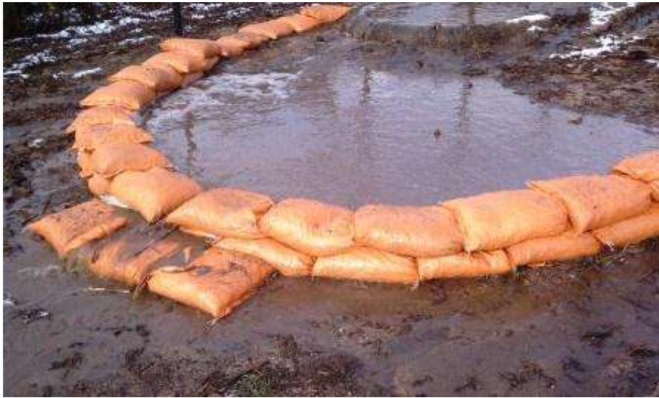
**Figure 11:** BMPs at Thing Valley Yard overrun with water during a storm event. (Link 2)
