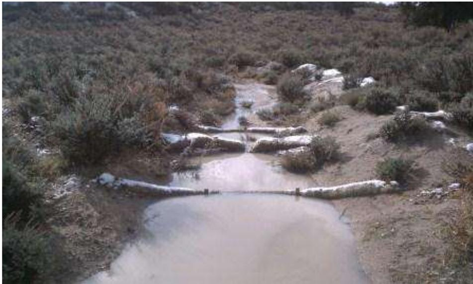
**Figure 5:** BMPs along La Posta Road overrun during a storm event.
