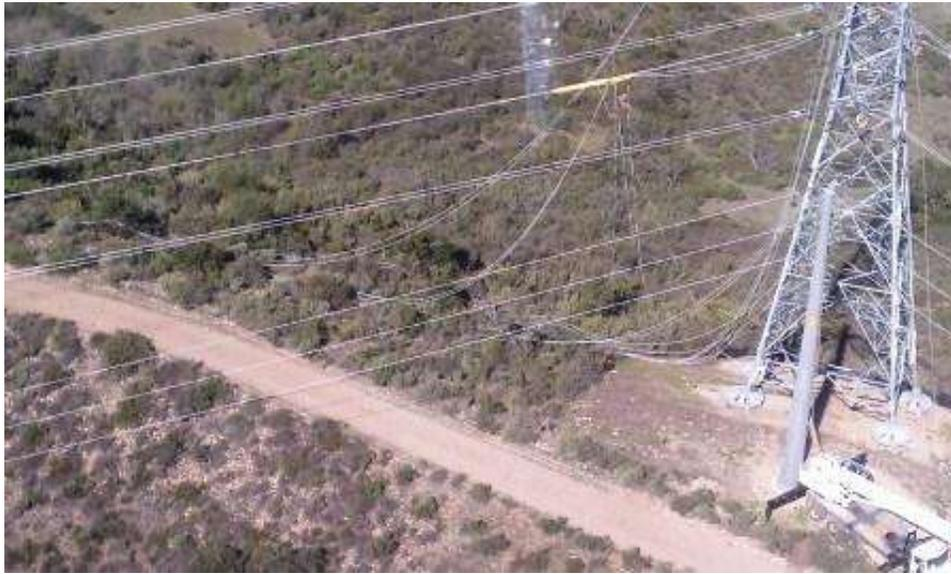
**Figure 5:** Conductor laid in brush at CP23. (Link 5)
