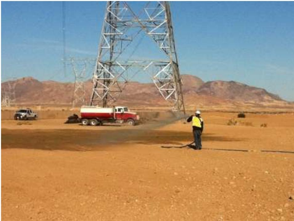
**Figure 10:** Tackifier and hydromulch application at Plaster City Yard. (Link 1)
