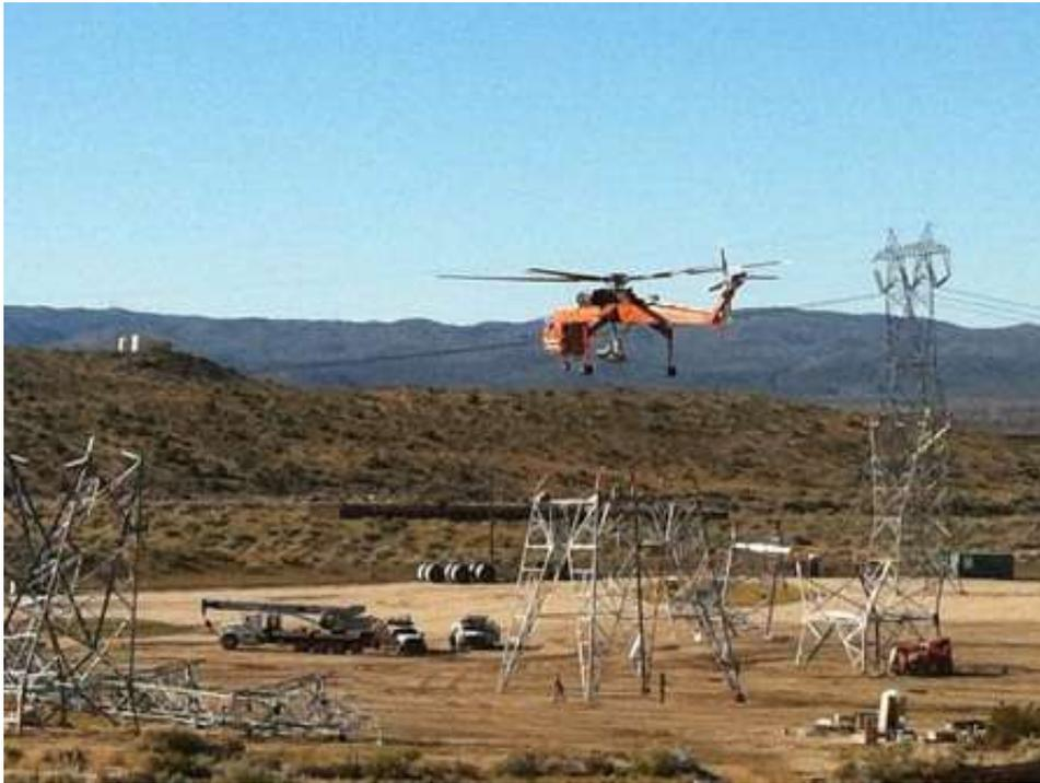
**Figure 3:** Aircrane “picking” a pre-assembled tower piece for Tower EP228.
