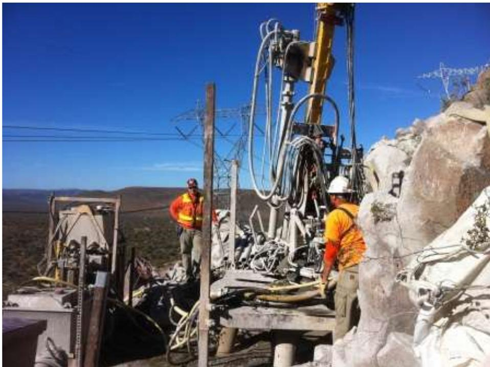
**Figure 2:** Micropile drilling at Tower EP254-3. (Link 1)
