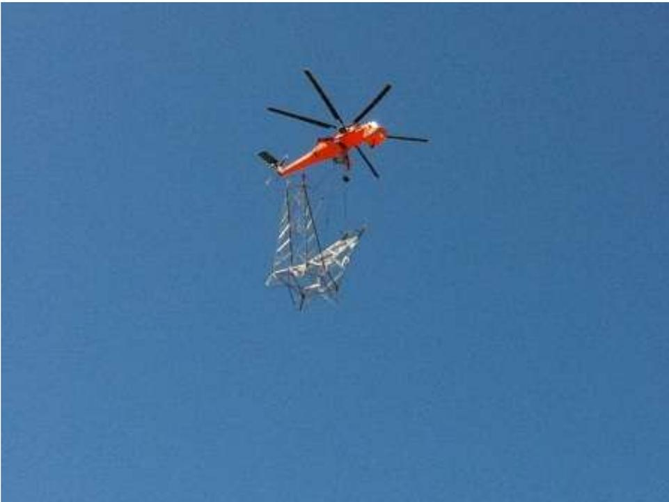
**Figure 2:** Air crane flying from JVR Yard to Tower EP252A-1 with pre-assembled tower piece. (Link 1)
