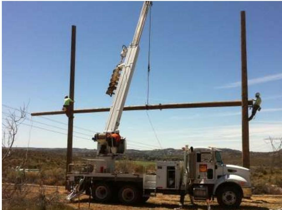
**Figure 4:** Guard pole installation over Carrizo Gorge Road, near Tower EP243. (Link 1)
