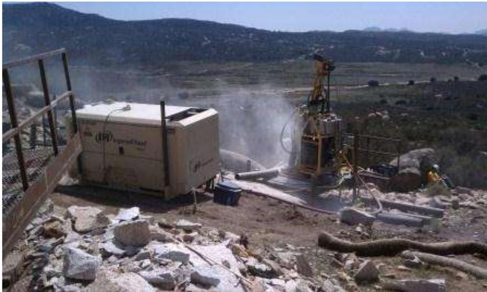
**Figure 8:** Micropile drilling at Tower EP64. (Link 2)
