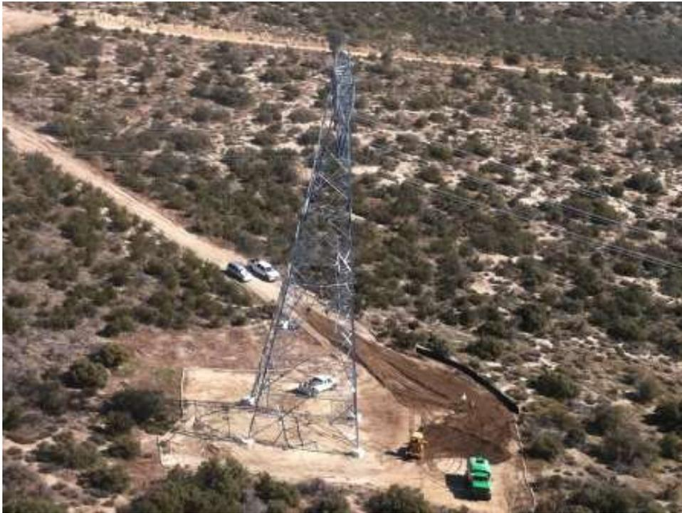
**Figure 7:** Final grading at Tower EP173-1. (Link 1)
