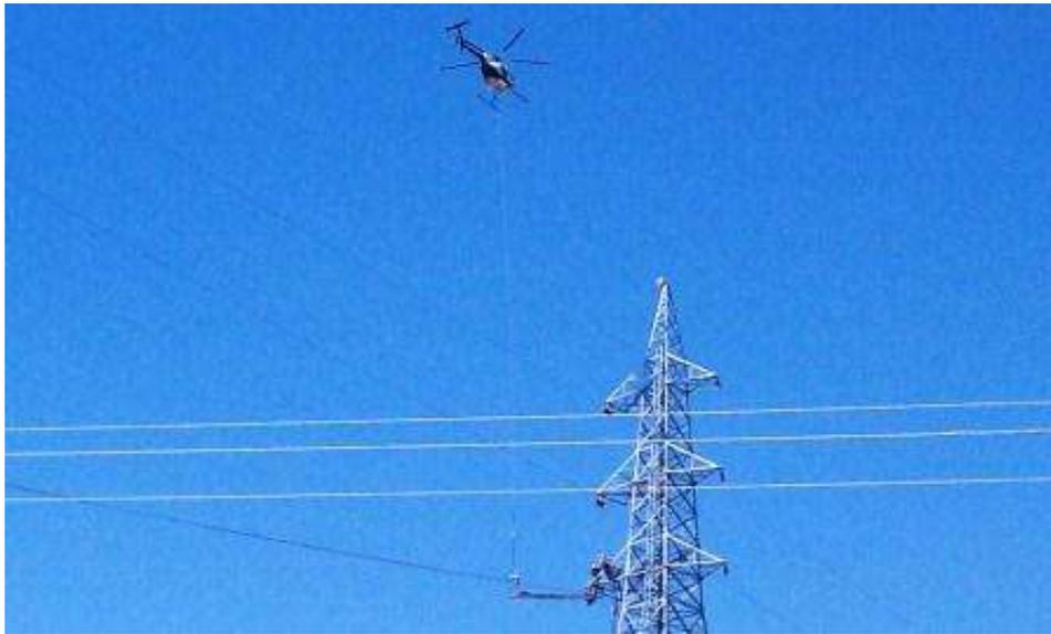
**Figure 9:** Helicopter hooking a platform at Tower CP43. (Link 5)
