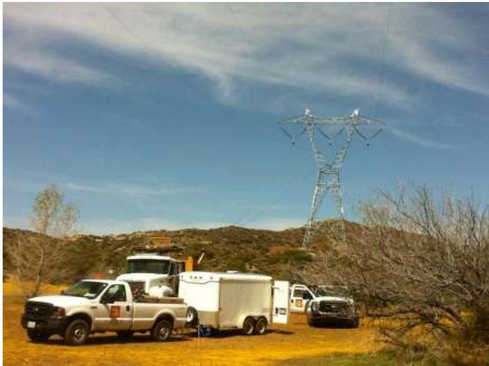
**Figure 6:** Utilizing a TEWS and pulling OPGW. (Link 1)
