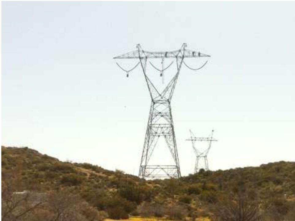
**Figure 5:** Traveler installation at Tower EP228. (Link 1)
