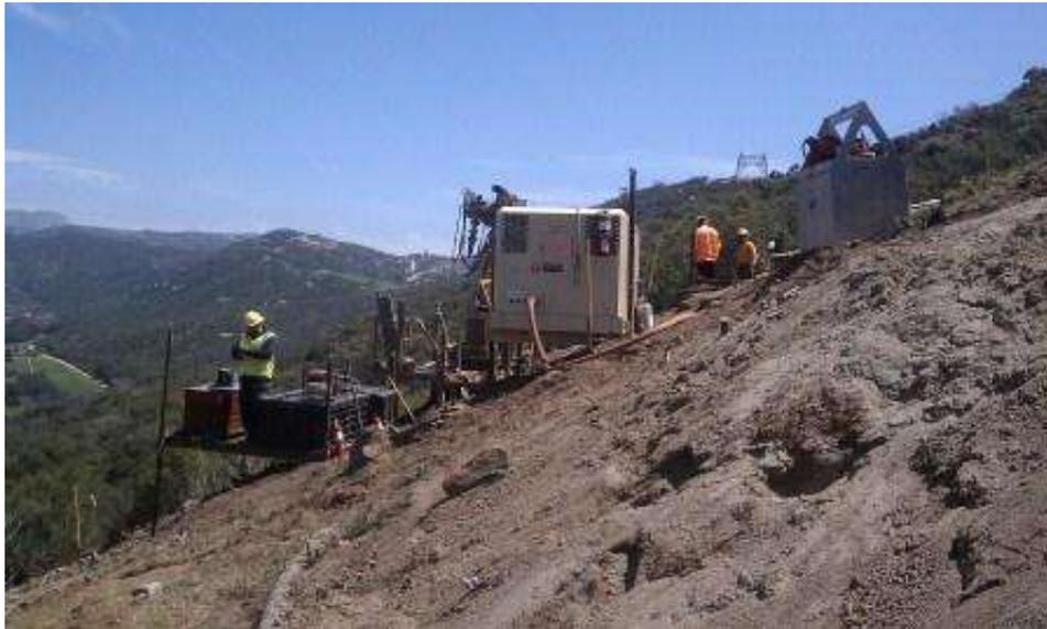
**Figure 5:** Micropile drilling at EP10-2. (Link 2)
