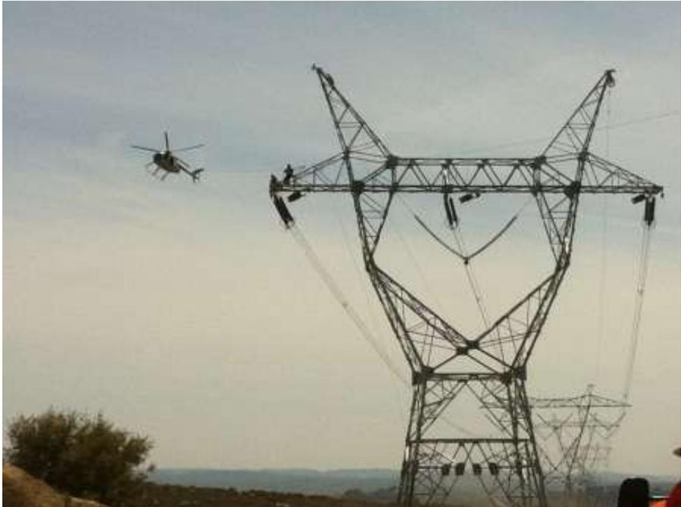
**Figure 2:** Flying sock line at Tower EP200-3. (Link 1)
