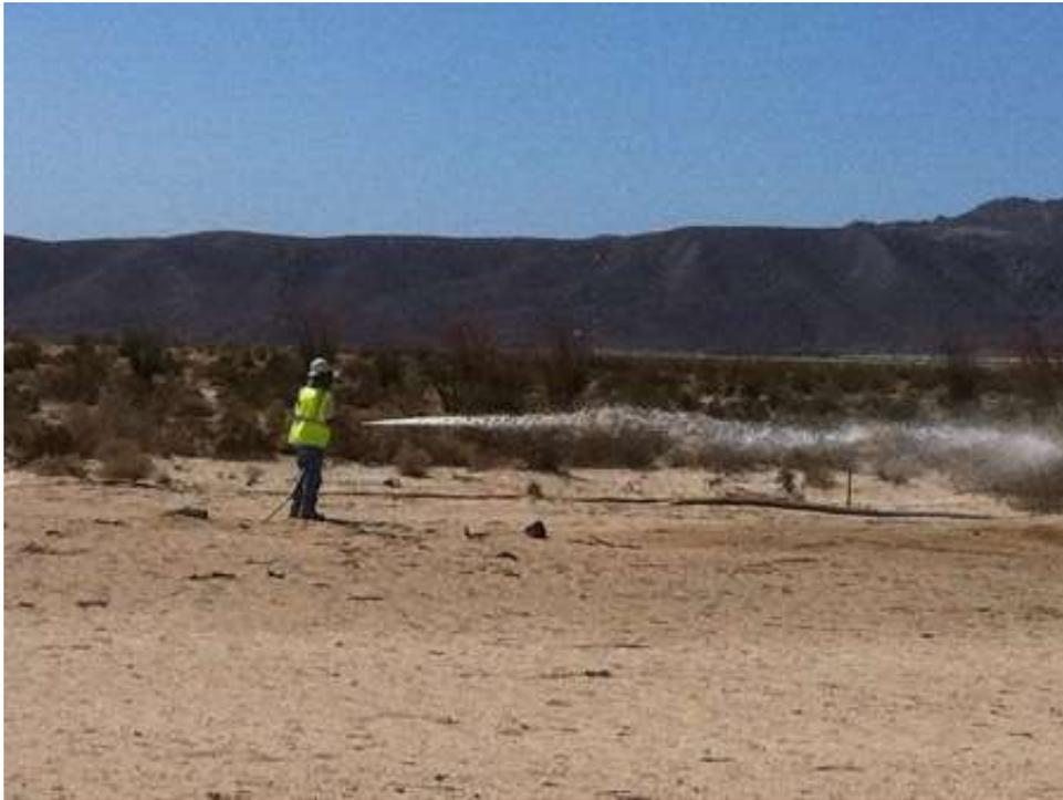
**Figure 11:** Applying tackifier to S2 Yard. (Link 1)
