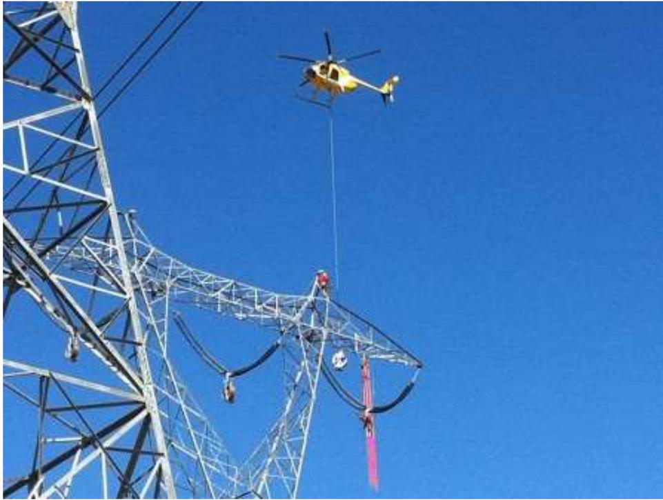
**Figure 1:** Travelers being installed at Tower EP253-2. (Link 1)
