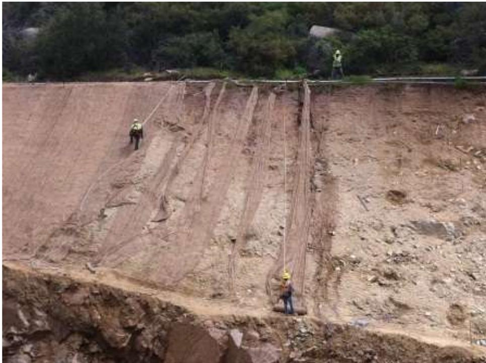
**Figure 8:** Jute installation along cut slopes at Suncrest Substation. (Link 3)
