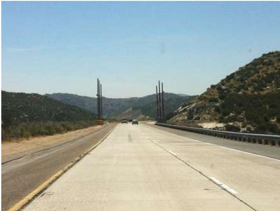
**Figure 4:** Guard structure installation over Interstate 8. (Link 2)
