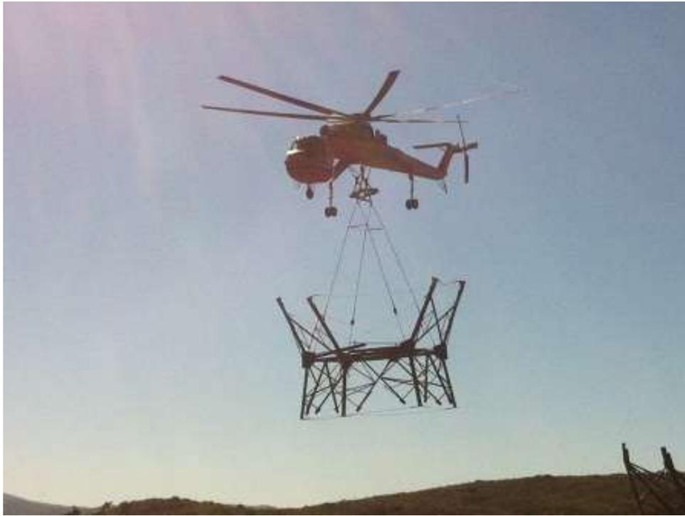
**Figure 5:** Air crane flying a tower section from Bartlett Hauser Yard.
