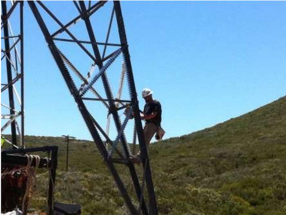
**Figure 1:** Installing anti-climbing guards at EP27-1. (Link 2)
