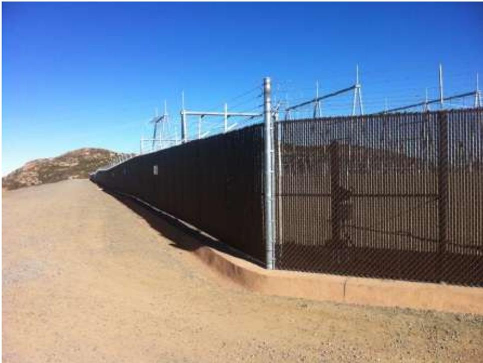
**Figure 2:** Fence slats installed along the southern side at Suncrest Substation. ([Link 3](#))
