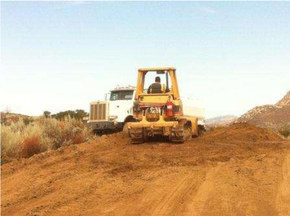
**Figure 2:** Final road grading at EP78-E to EP79-E-C. (Link 2)
