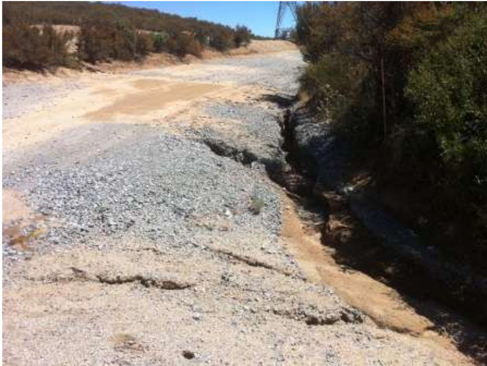
**Figure 7:** Gully created by significant rain event along La Posta Truck Trail near EP124/EP125 pull site. (Link 2)
