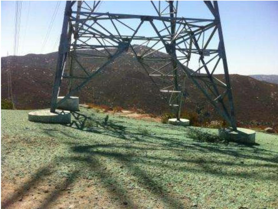
**Figure 5:** Hydromulching at Tower CP100-1. (Link 5)
