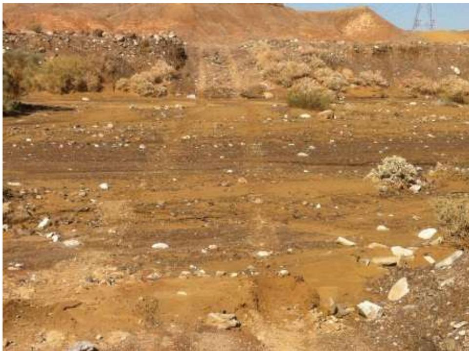
**Figure 8:** Southwest Power Line (SWPL) road wash-out due to flooding in the desert near Tower EP316. (Link 1)
