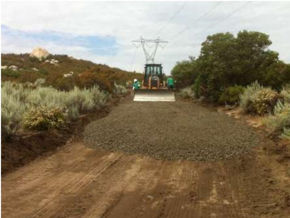
**Figure 3:** Final road grade and placing Class 2 base on access road between EP112A-1 and EP113-5. (Link 2)
