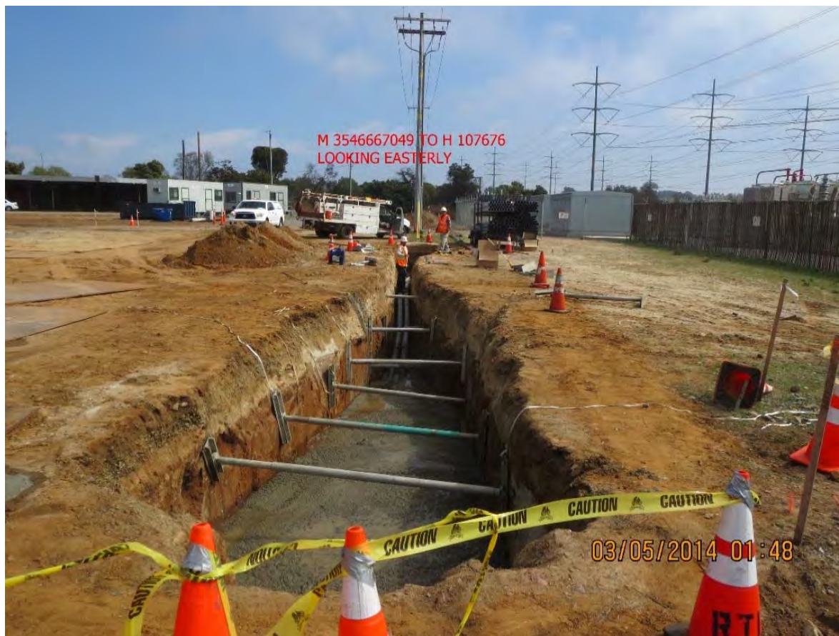
A. Typical 12-kV Trench
