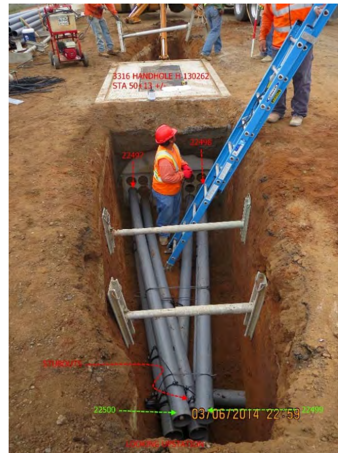
B. Typical 12-kV Duct Bank
