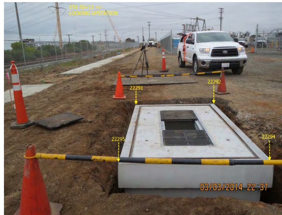
D. Typical Vault Installation
