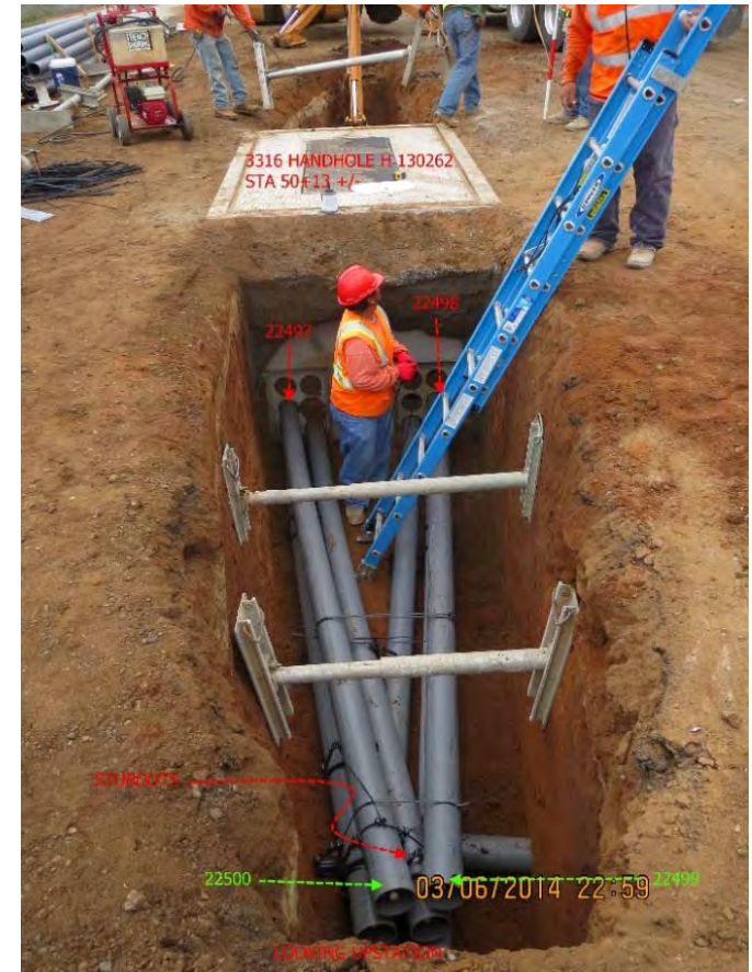
B. Typical 12-kV Duct Bank
