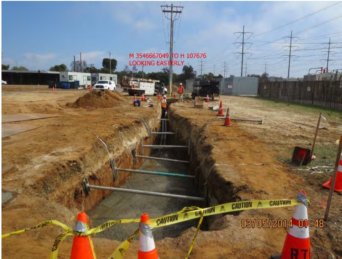
A. Typical 12-kV Trench
