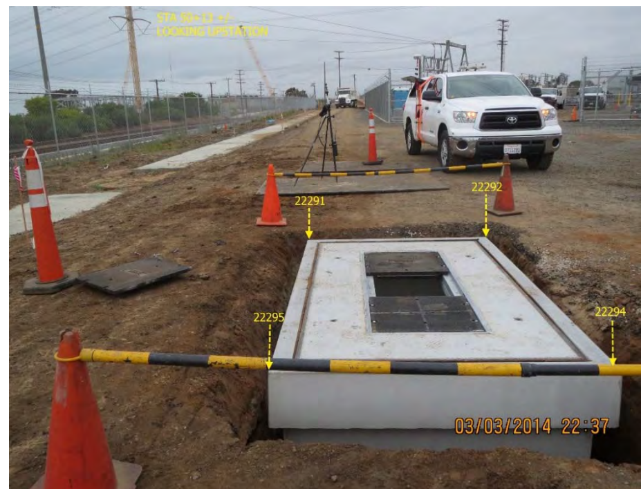
D. Typical Vault Installation
