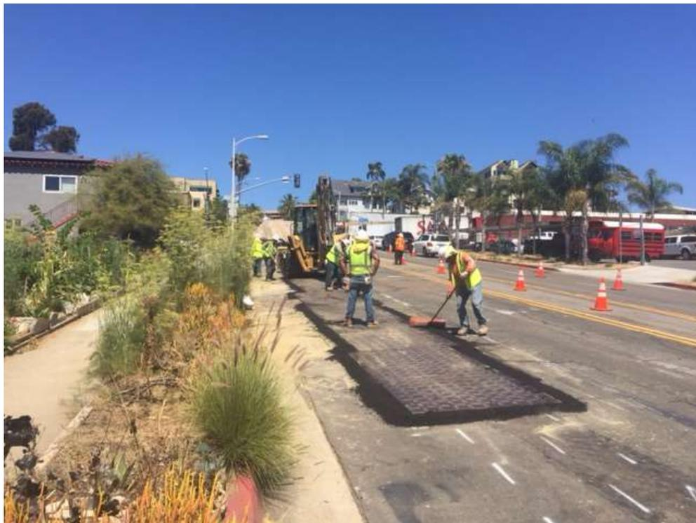
Figure 2 – Steel plate placement over the trenchline at the end of the day along Laurel Street.
