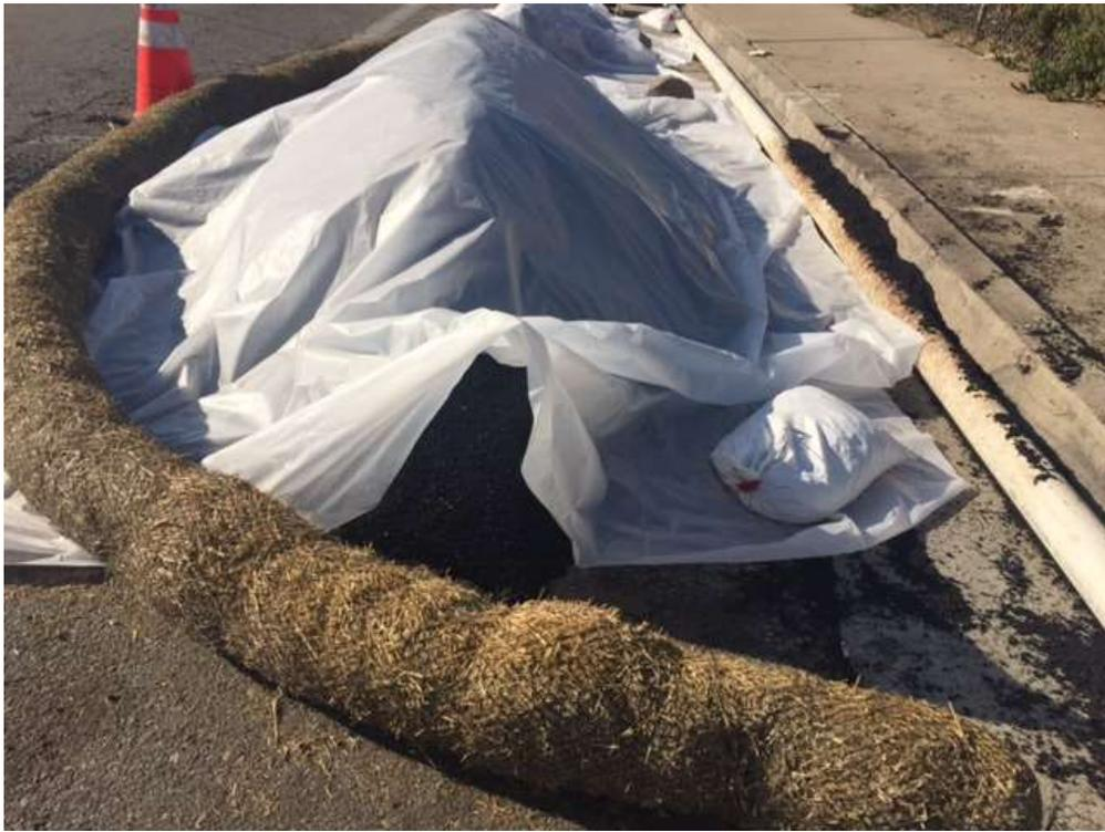
Figure 6 – Cold mix stored directly on the street along Columbia Street.
