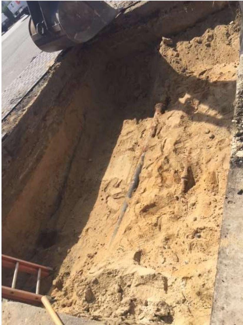
Figure 3 – Abandoned utility pipes found during vault excavations along Columbia Street.
