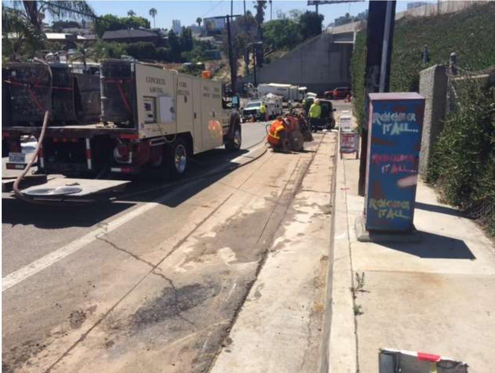
Figure 1 – Crews saw-cutting along Columbia Street in advance of trenching crews.
