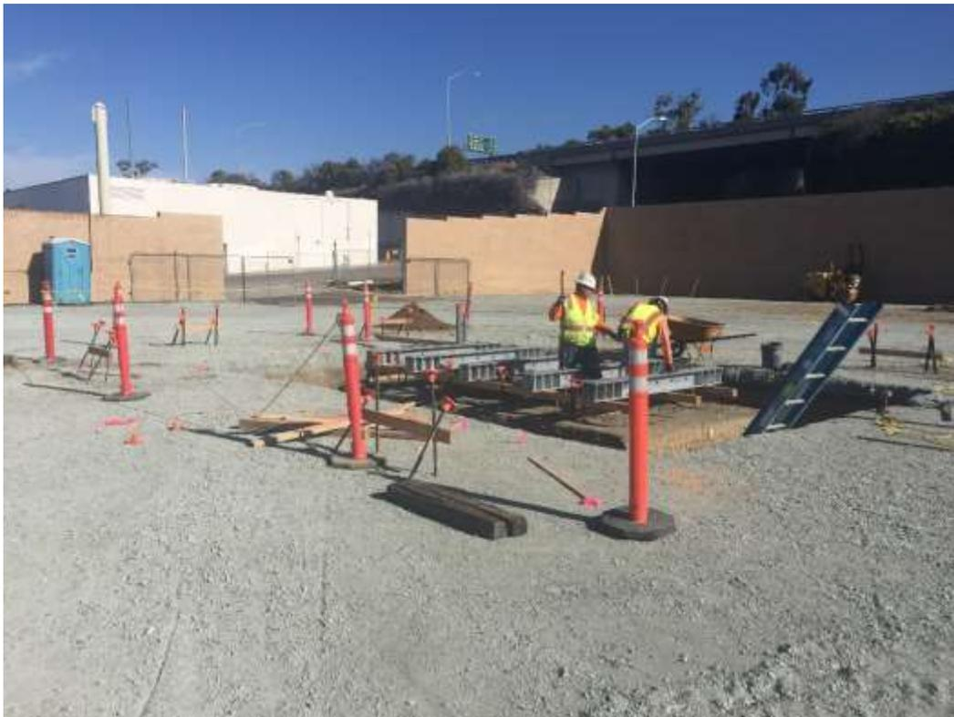
Figure 4 – DCX crews installing steel at one of the transformer pads within the substation, February 15, 2017.
