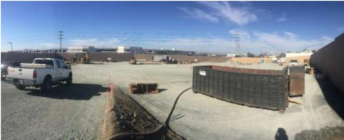
Figure 2 – Rock base has been placed throughout the interior of the substation, February 15, 2017.
