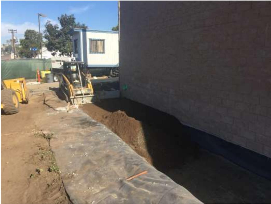
Figure 3 – Bio-retention swale liner and aggregate installation immediately outside of the perimeter wall boundary, February 15, 2017.
