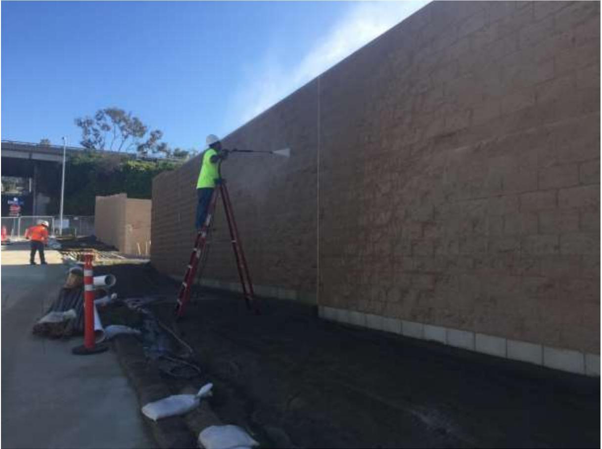
Figure 1 – Patriot crews preparing the perimeter block wall for anti-graffiti treatment, February 15, 2017.
