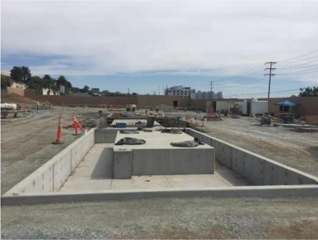
Figure 1 – DCX crews constructed the oil containment area surrounding the transformer pads.
