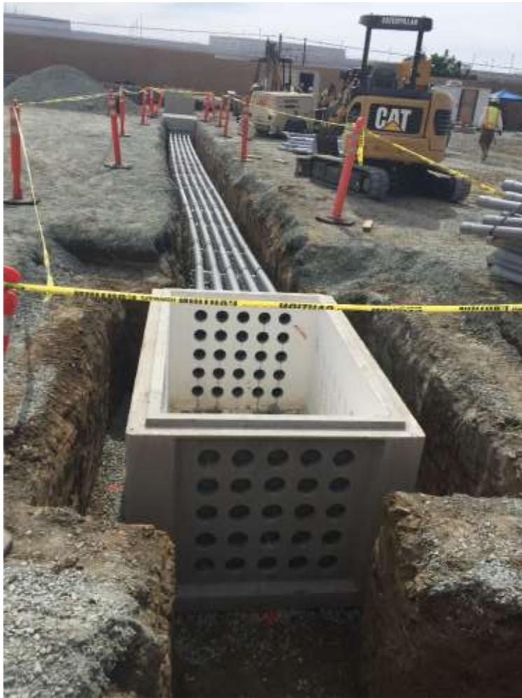
Figure 3 – Conduit and pull box installation is ongoing.
