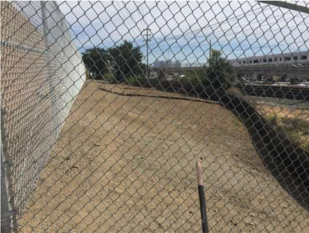
Figure 5 – Temporarily disturbed area adjacent to the railroad right-of-way; SDG&E is assessing possible stabilization treatments.
