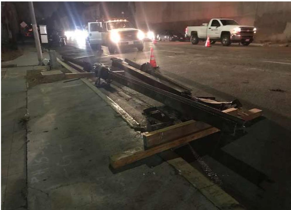
Figure 2 – NPL crews working along Kettner Boulevard encountered abandoned rail segments. These sections are put aside for recycling and for collection by the Pacific Southwest Railway Museum.
