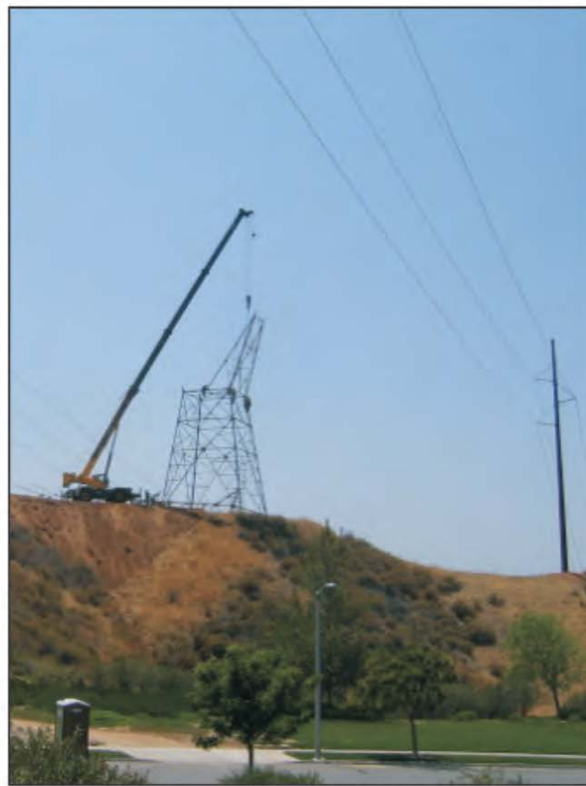
Photo 2. Shoo-fly in use during 220 kV tower removal.
