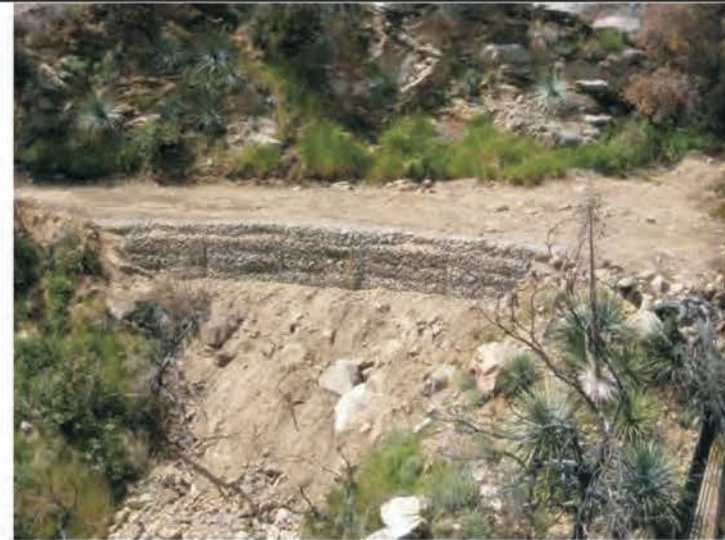
Typical gabion wall.
