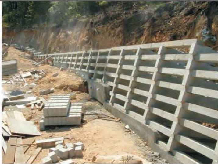
Typical concrete crib wall.
