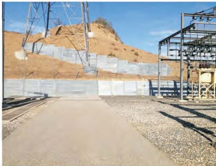
Typical soldier pile wall.
