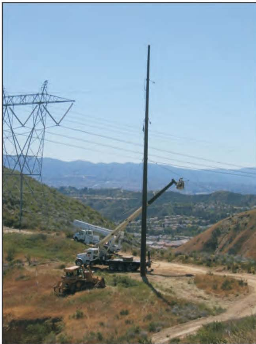
Photo 1. Wire installation on a shoo-fly pole.
